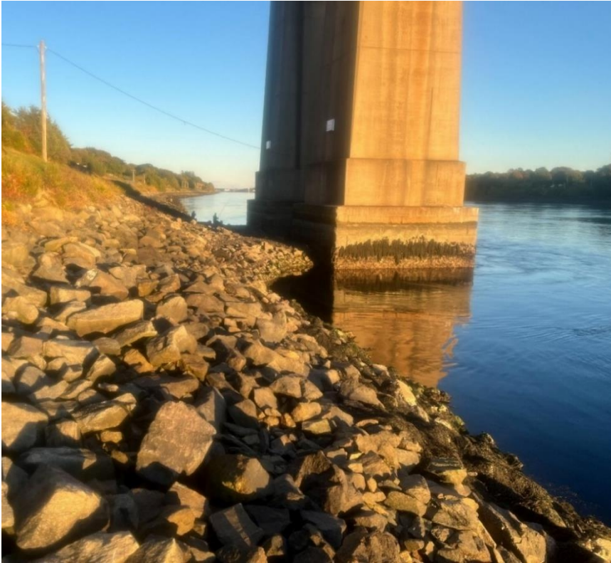
Exhibit 5-1. Banks of Cape Cod Canal Adjacent to Sagamore North Quadrant Bridge Piers, Looking East
