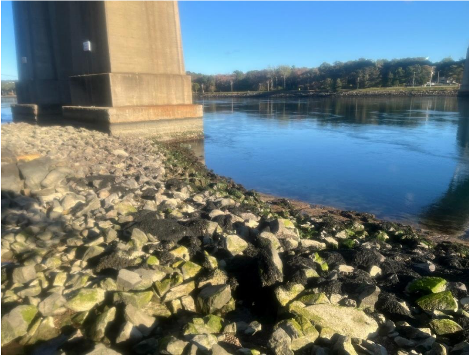
Exhibit 5-5. Banks of Cape Cod Canal Adjacent to Bourne North Quadrant Bridge Piers, Looking East
