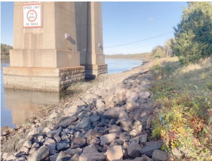
Exhibit 5-8. Banks of Cape Cod Canal Adjacent to Bourne South Quadrant Bridge Piers, Looking East (closeup view)
