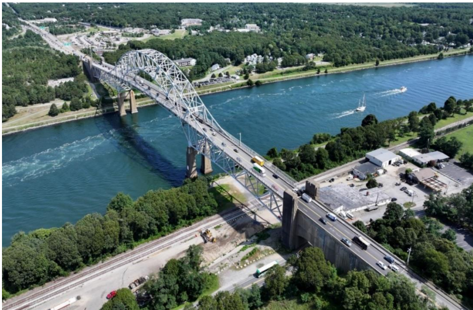
Exhibit 1-1. Aerial View of Sagamore Bridge (looking north)
