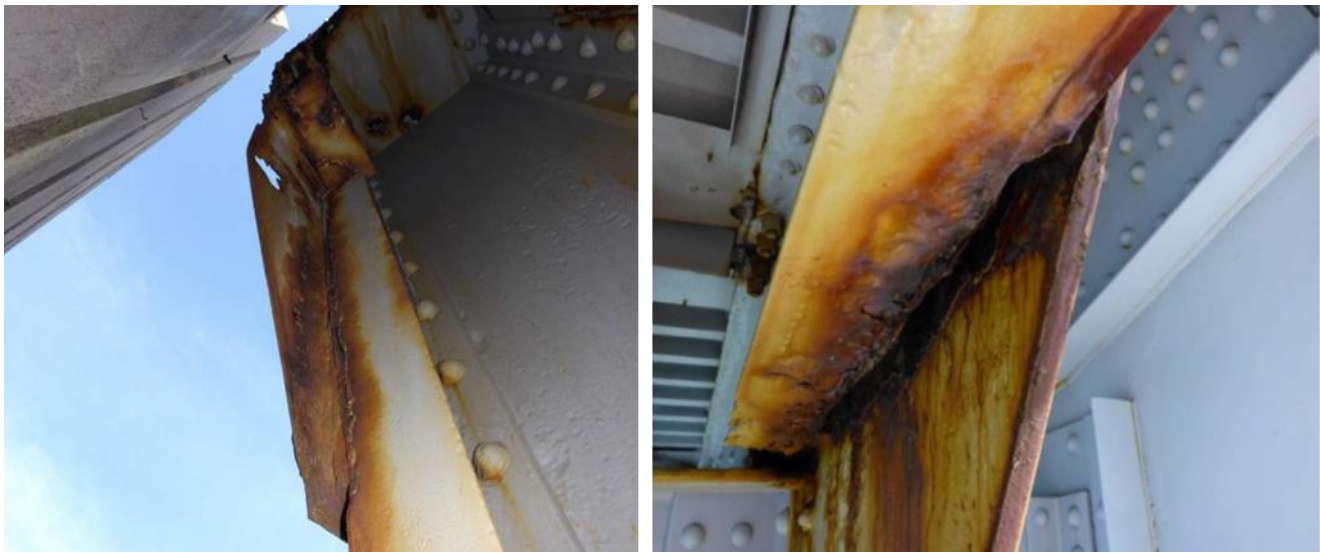
Exhibit 2-1. Truss Joint Gusset Plate Deterioration (Sagamore Bridge)
