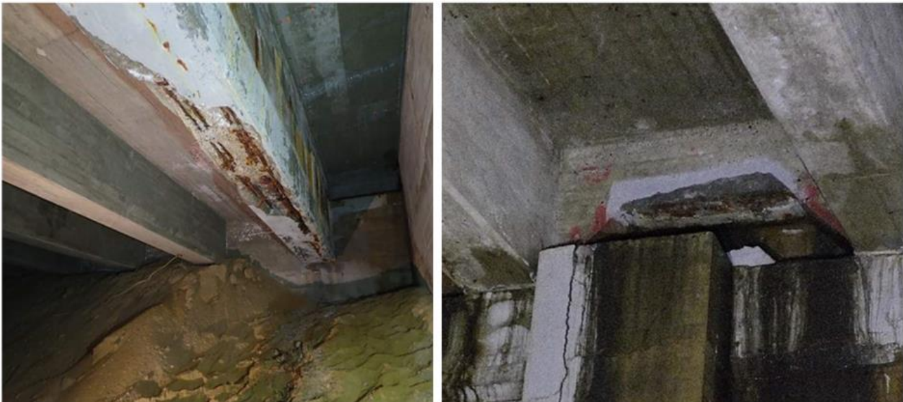
Exhibit 2-3. Concrete T-Beam Deterioration (Bourne Bridge)
