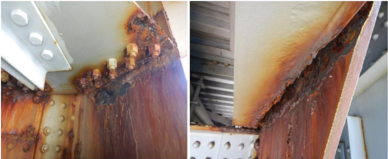
Exhibit 2-2. Truss Joint Gusset Plate Deterioration (Bourne Bridge)
