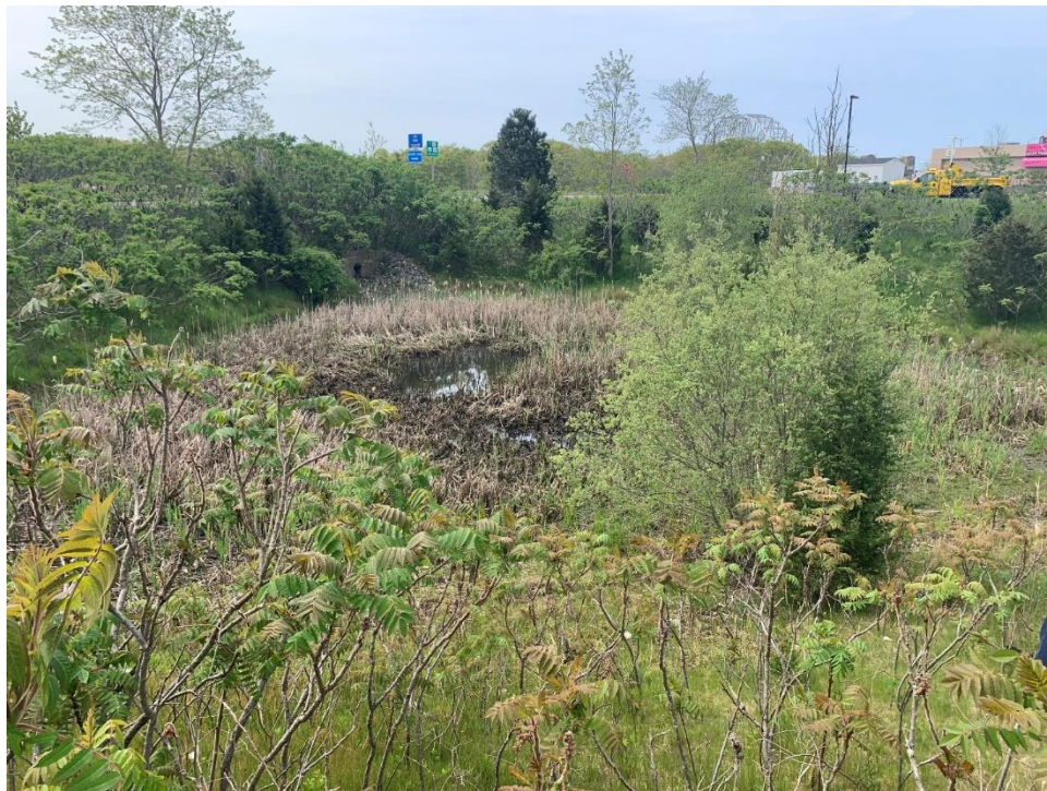
Exhibit 4.10-2. Stormwater Basin at Canal Street and Commerce Way (Sagamore North Quadrant)
