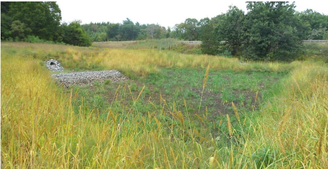
Exhibit 4.10-8. Typical Infiltration Basin with Sediment Forebay
