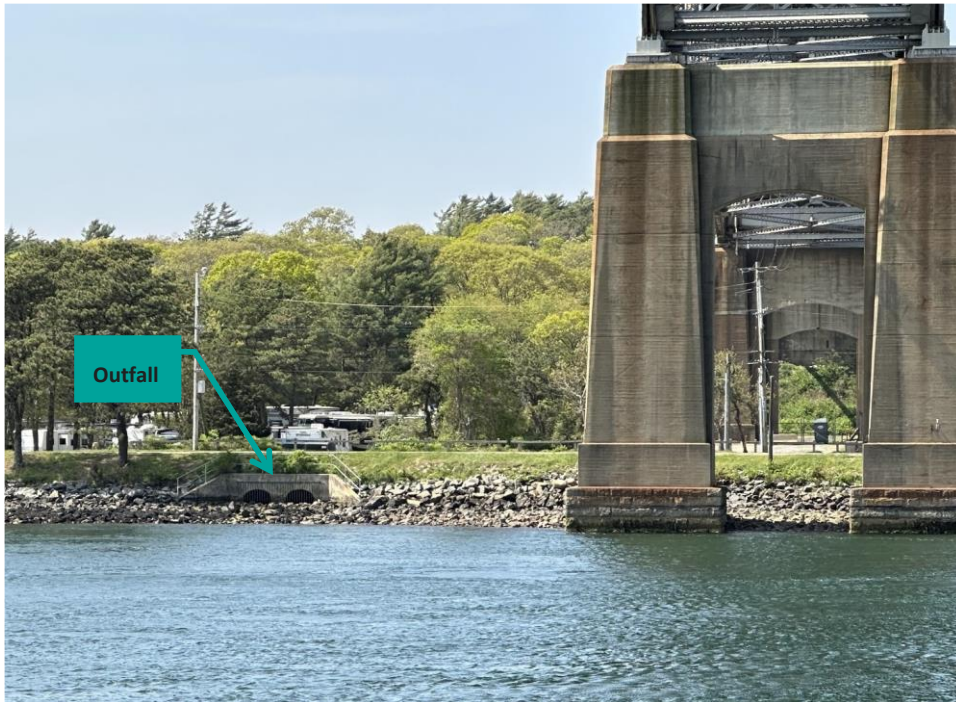
Exhibit 4.10-4. Pipe Outfall Location at Cape Cod Canal (Bourne North Quadrant)
