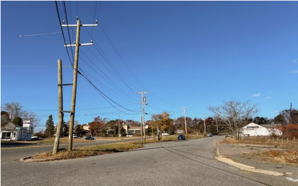
Exhibit 4.15-10a. Existing View from Cranberry Highway at Adams Street, facing west
