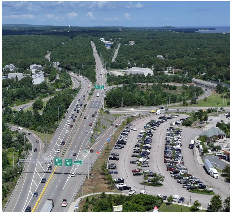
Exhibit 4.2-1. Aerial View of Bourne Park and Ride Lot, facing north, August 2024
