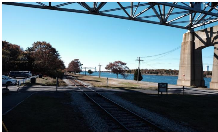
Exhibit 4.2-2. Cape Main Line Railroad Track under Bourne Bridge, October 2024
