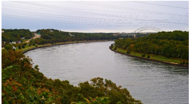
Exhibit 4.4-1. View of Cape Cod Canal, facing west toward Sagamore Bridge, September 2023
