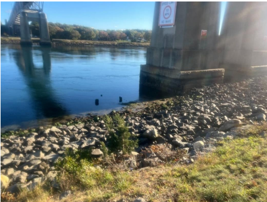
Exhibit 4.9-6. Banks of Cape Cod Canal Adjacent to Bourne North Quadrant Bridge Piers, Looking South
