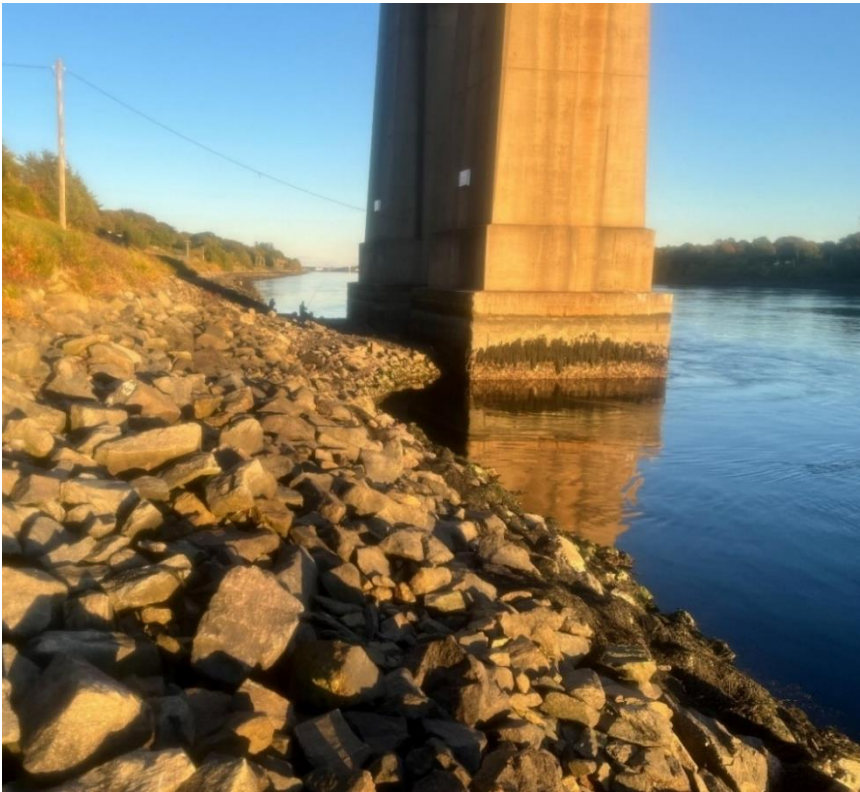
Exhibit 4.9-1. Banks of Cape Cod Canal Adjacent to Sagamore North Quadrant Bridge Piers, Looking East
