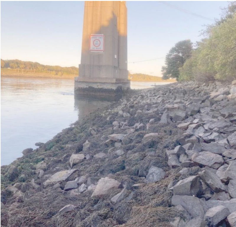
Exhibit 4.9-3. Banks of Cape Cod Canal Adjacent to Sagamore South Quadrant Bridge Piers, Looking East
