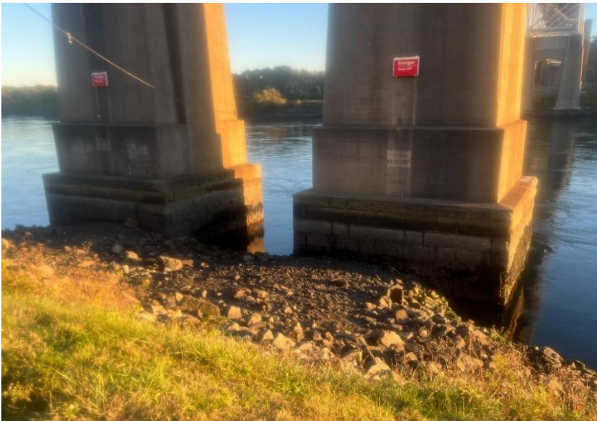
Exhibit 4.9-2. Banks of Cape Cod Canal Adjacent to Sagamore North Quadrant Bridge Piers, Looking South
