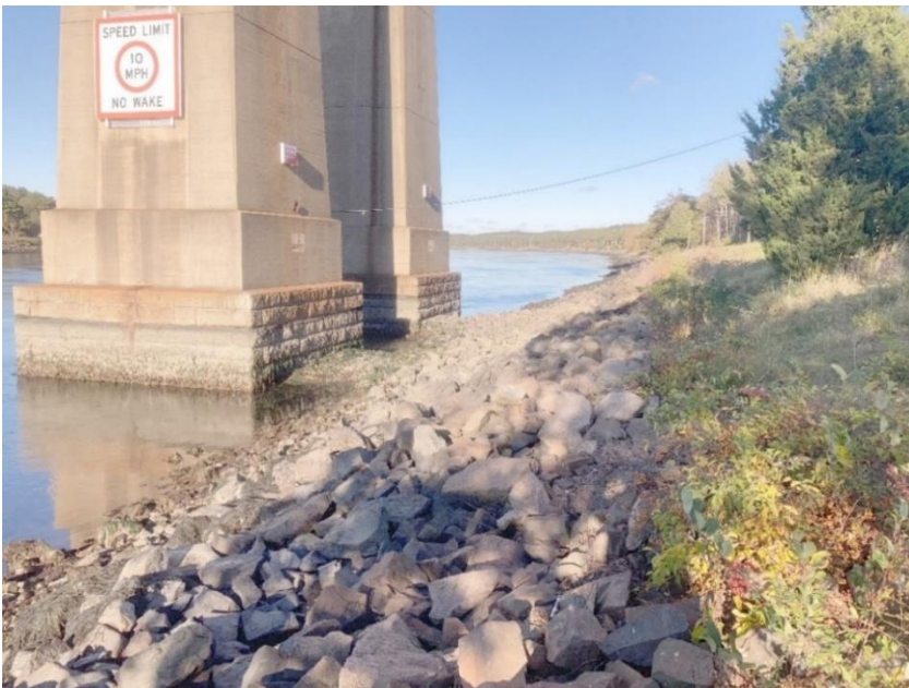
Exhibit 4.9-8. Banks of Cape Cod Canal Adjacent to Bourne South Quadrant Bridge Piers, Looking East (closeup view)
