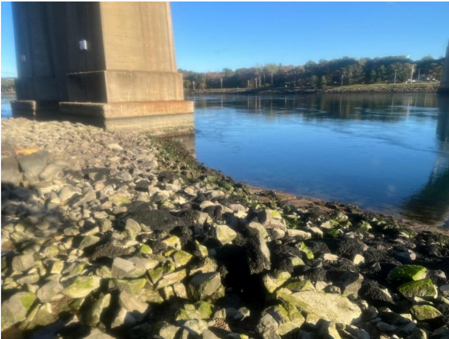
Exhibit 4.9-5. Banks of Cape Cod Canal Adjacent to Bourne North Quadrant Bridge Piers, Looking East
