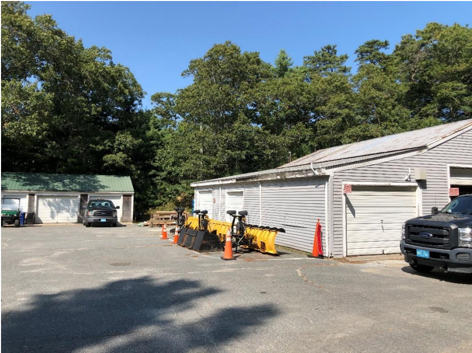
Exhibit 5-12. Bourne Scenic Park: Maintenance Buildings, facing northeast
