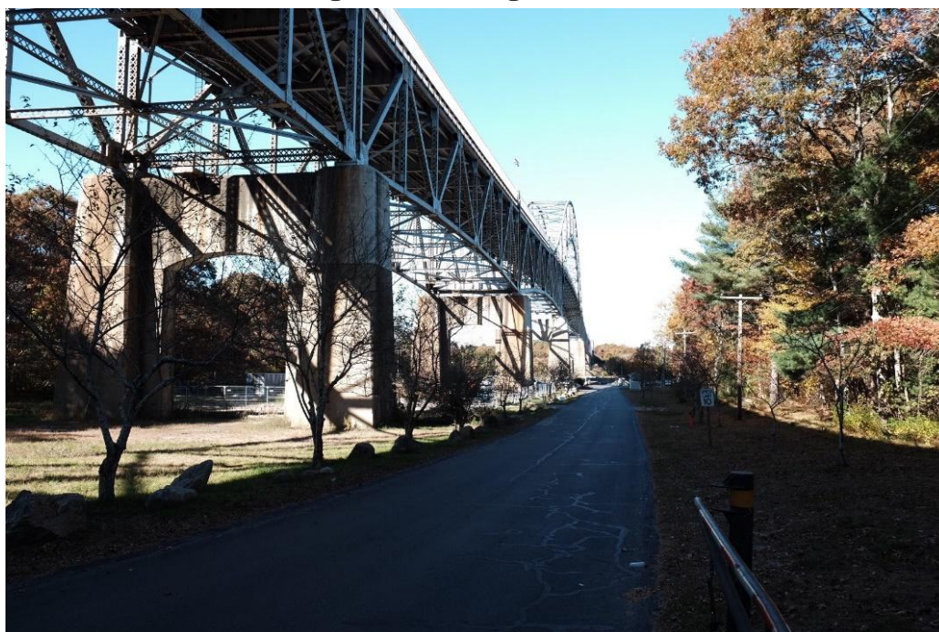
Exhibit 5-24. Bourne Bridge Road, facing north from Sandwich Road
