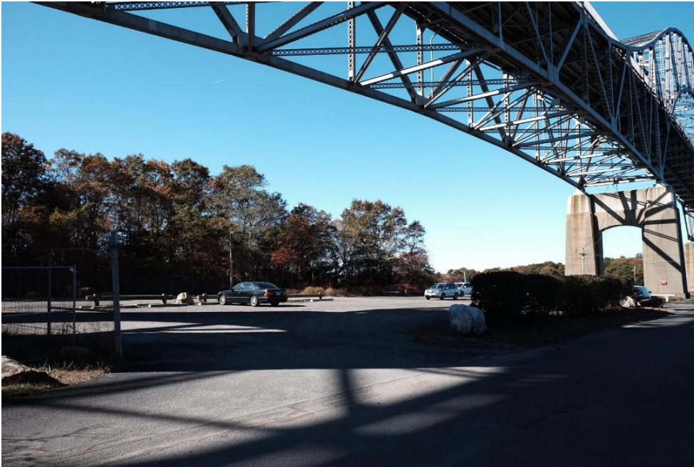
Exhibit 5-25. Overflow Gravel Parking Area, facing northwest from Bourne Bridge Road
