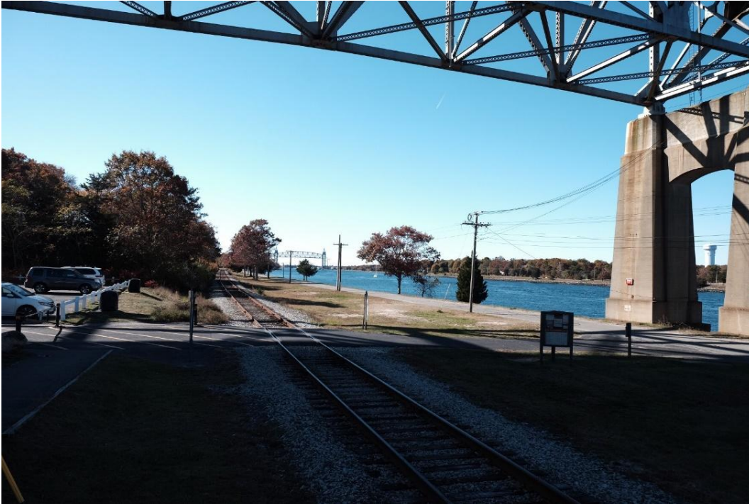
Exhibit 5-27. Cape Cod Railroad Tracks, facing east at Bourne Bridge (outside of Bourne Recreation Area)
