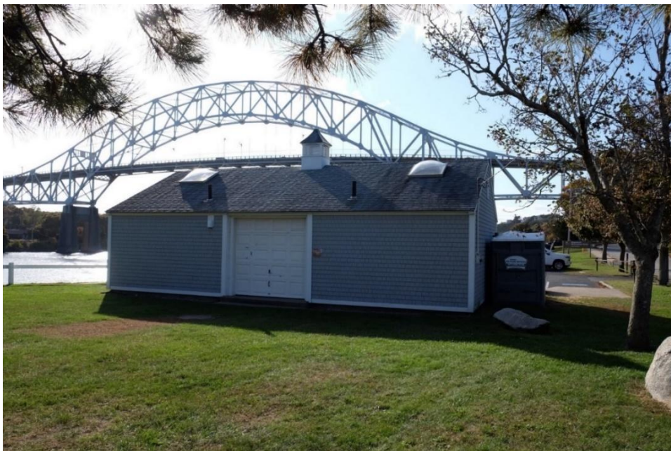
Exhibit 5-2. Sagamore Recreation Area: Seasonal Comfort Station and Portable Toilets, facing west
