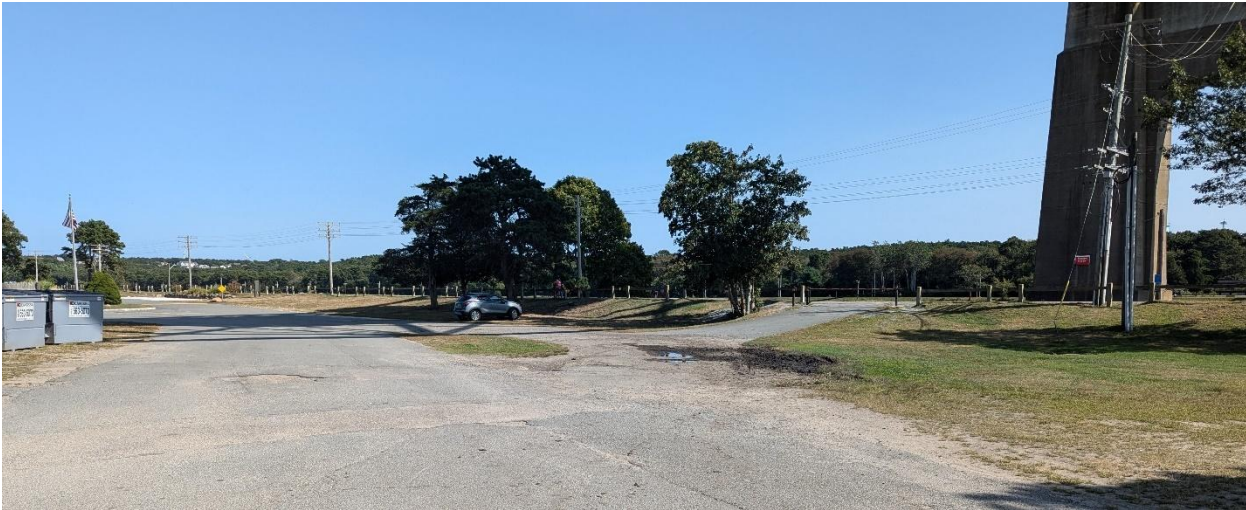
Exhibit 5-20. Access to North Canal Service Road at Bourne Bridge abutment, facing south
