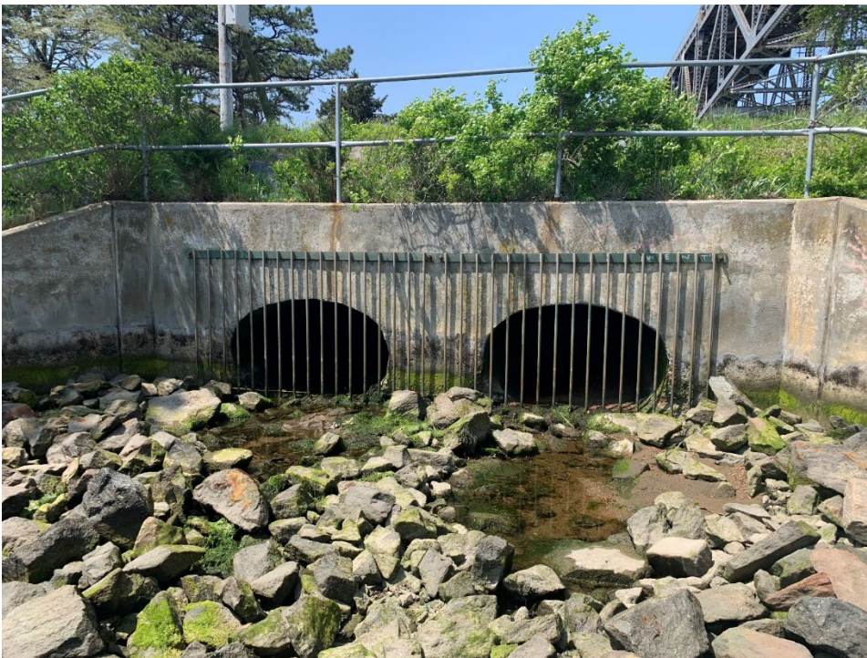
Exhibit 5-5. Twin 43-inch by 68-inch Elliptical Pipe Outfalls (Bourne North Quadrant)
