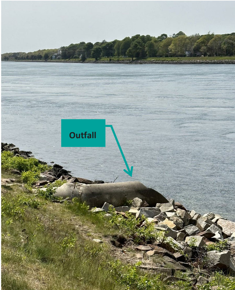
Exhibit 5-6. 24-Inch Pipe Outfall at Cape Cod Canal (Bourne South Quadrant)
