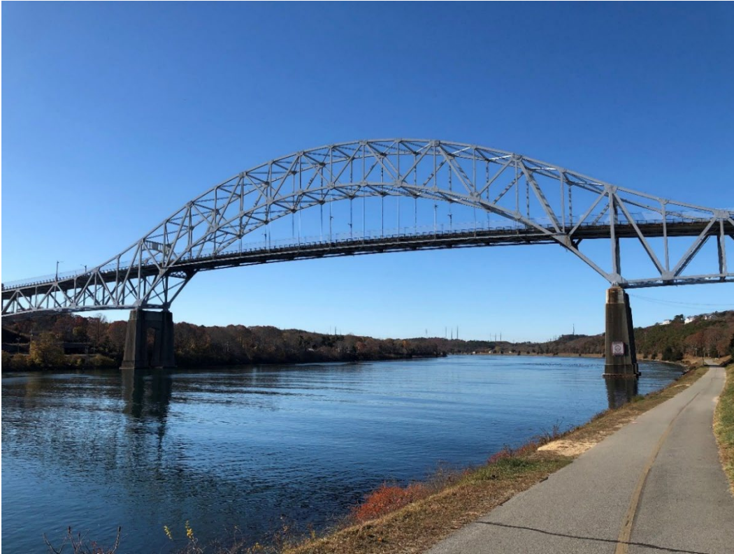
Exhibit 7-2a. Existing View of Sagamore Bridge or Bourne Bridge from Canal Service Road
