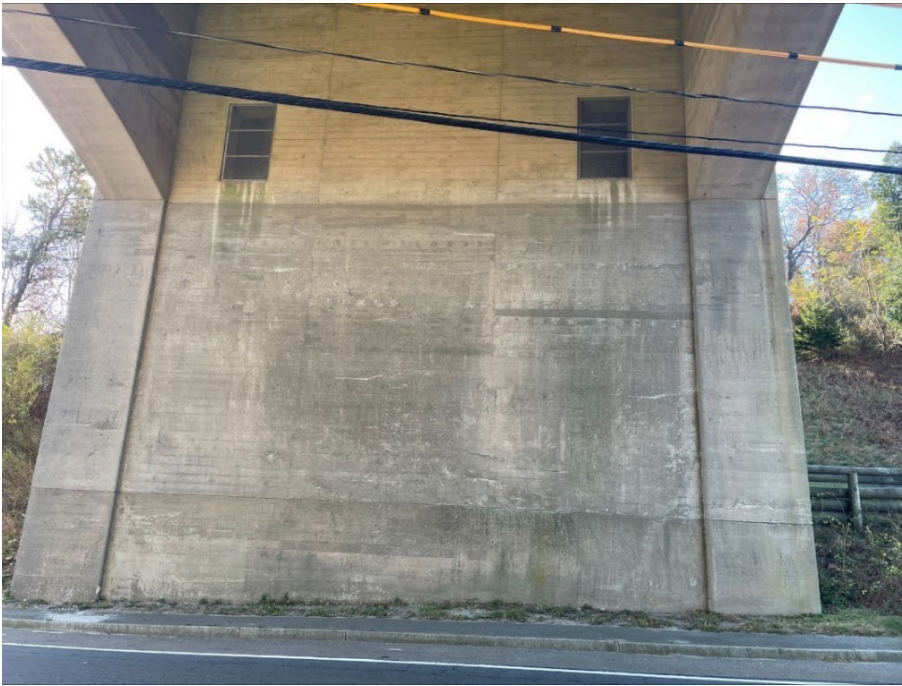
Exhibit 7-10a. Existing View of Sagamore Bridge South Abutment from Sandwich Road, facing south
