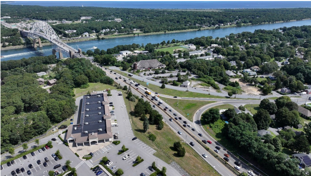
Exhibit 6-7. U.S. Route 6 facing northwest to Sagamore Bridge (Sagamore South Quadrant)
