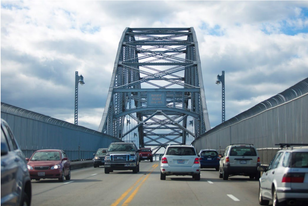
Exhibit 7-1a. Existing View of Bridge Arch from Motorist (Sagamore and Bourne Bridges)
