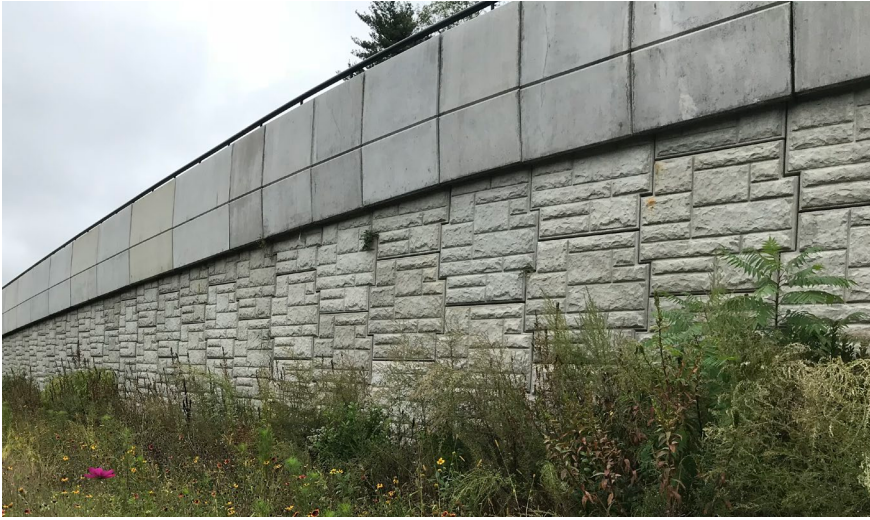
Exhibit 8-6. Example of Low Exposure Prefabricated Wall System
