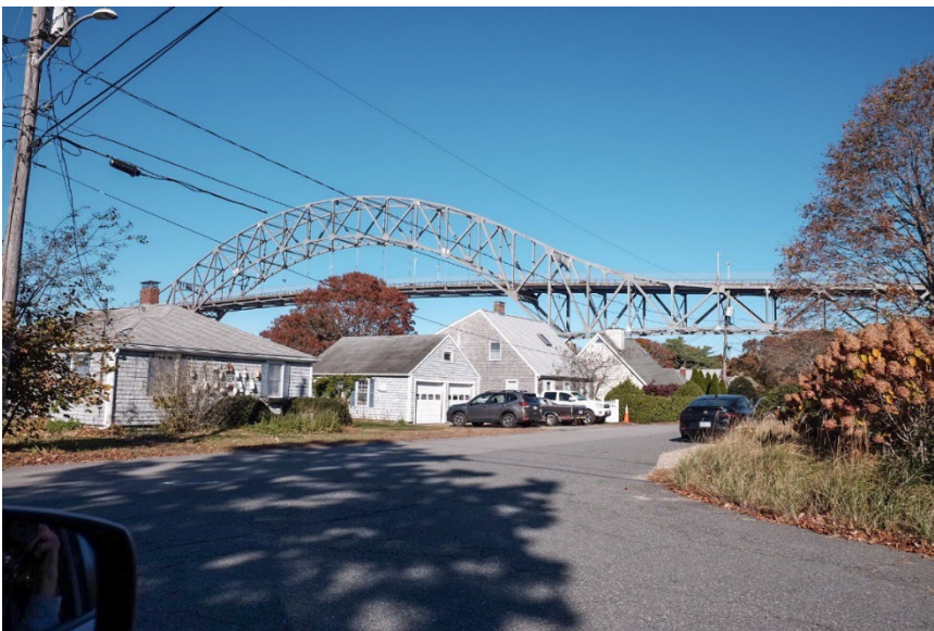
Exhibit 6-13. View of Bourne Bridge from Winslow Street, facing northeast
