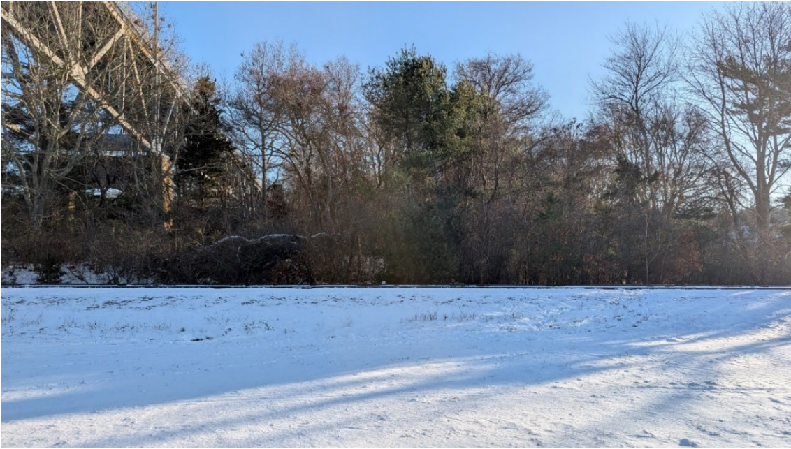
Exhibit 7-19a. Existing View of Bourne Bridge from South Canal Service Road, facing south
