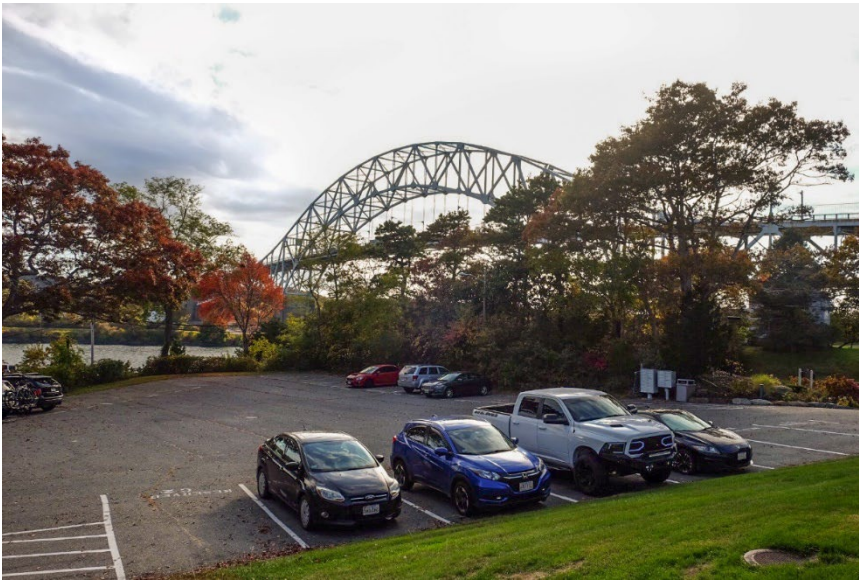
Exhibit 6-12. View of Sagamore Bridge from Hunters Brook Condominiums, facing southwest
