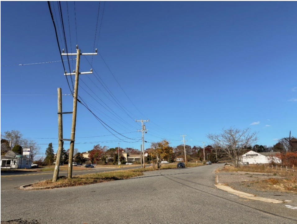
Exhibit 7-11a. Existing View of Cranberry Highway at Adams Street, facing west
