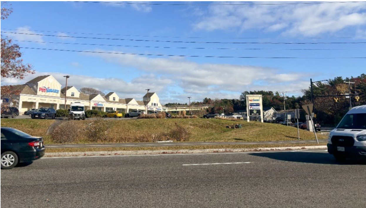
Exhibit 7-12a. Existing View of State Route 25 from Belmont Circle, facing east
