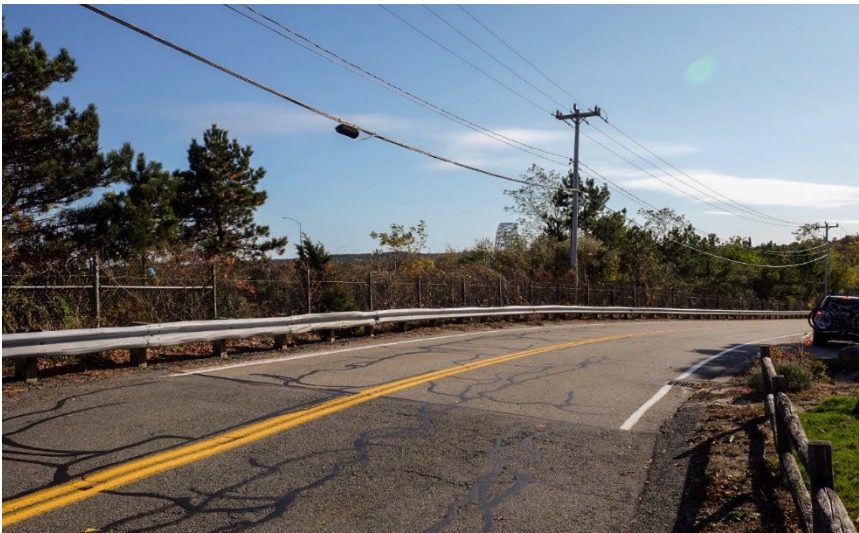
Exhibit 6-10. View of Sagamore Bridge from Church Lane at Cape Pine Road, facing south
