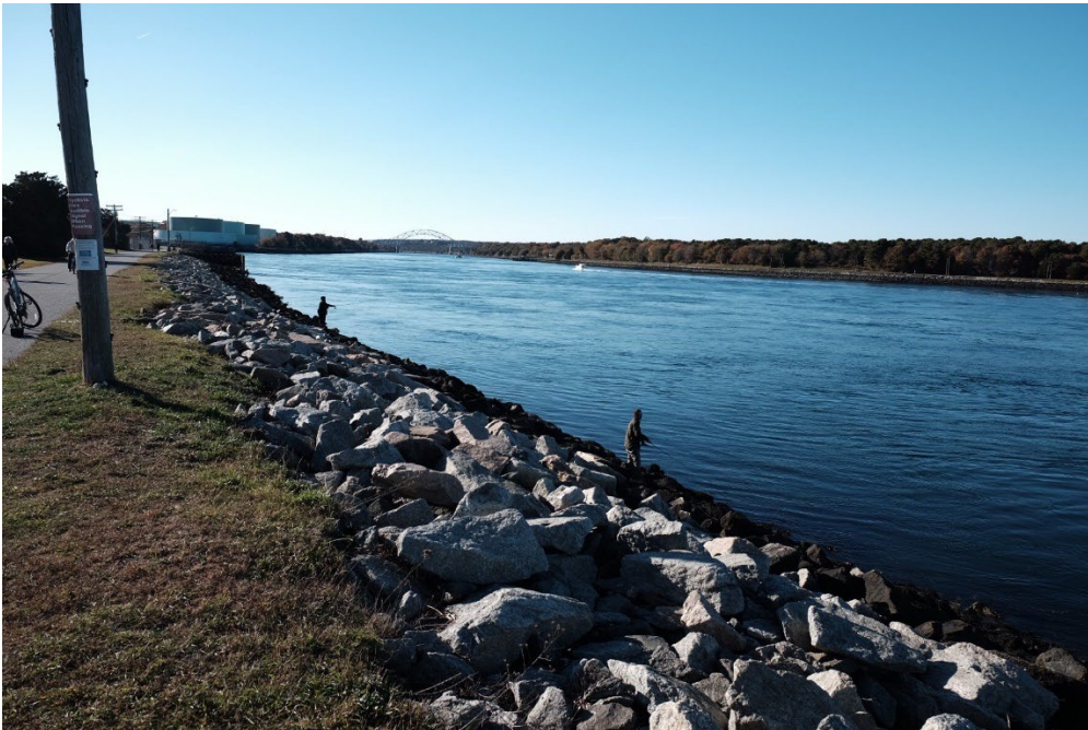
Exhibit 5-4. View of Cape Cod Canal Historic District, facing northwest
