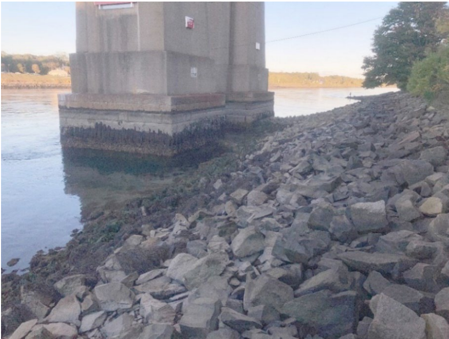
Exhibit 5-4. Banks of Cape Cod Canal Adjacent to Sagamore South Quadrant Bridge Piers, Looking East-Northeast
