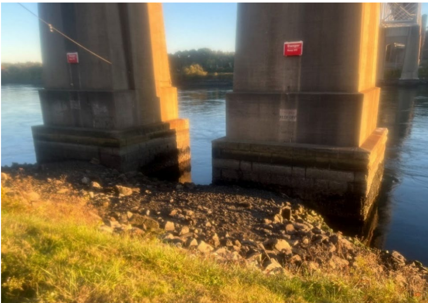
Exhibit 5-2. Banks of Cape Cod Canal Adjacent to Sagamore North Quadrant Bridge Piers, Looking South
