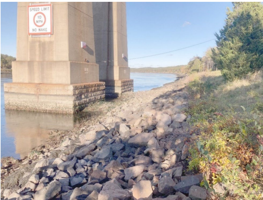
Exhibit 5-8. Banks of Cape Cod Canal Adjacent to Bourne South Quadrant Bridge Piers, Looking East (closeup view)
