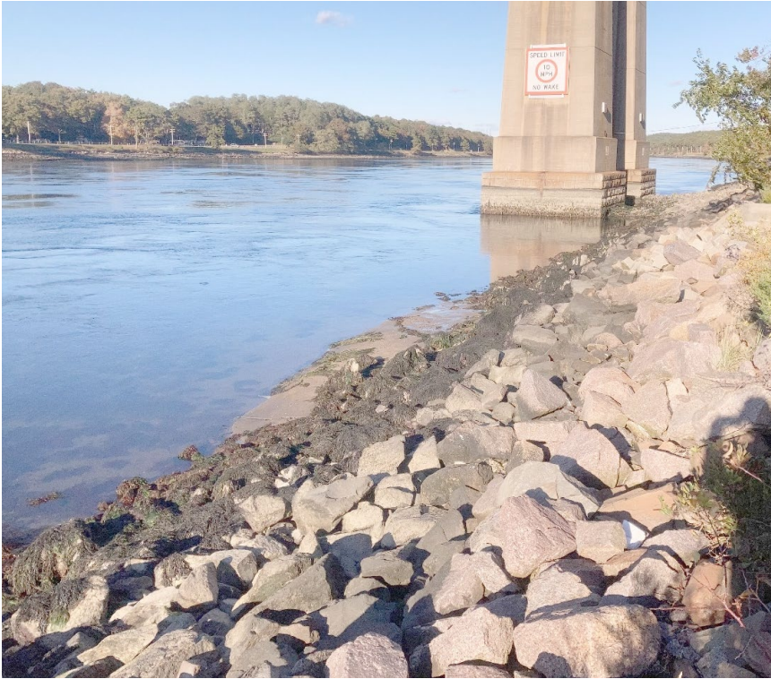
Exhibit 5-7. Banks of Cape Cod Canal Adjacent to Bourne South Quadrant Bridge Piers, Looking East
