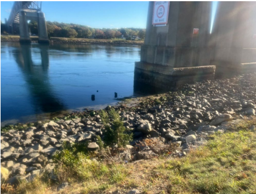
Exhibit 5-6. Banks of Cape Cod Canal Adjacent to Bourne North Quadrant Bridge Piers, Looking South
