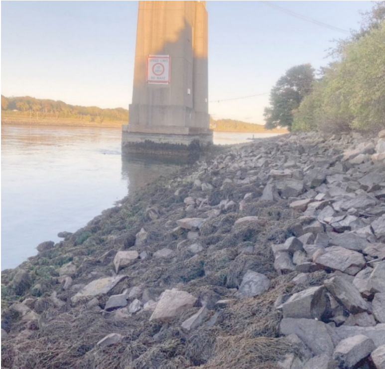
Exhibit 5-3. Banks of Cape Cod Canal Adjacent to Sagamore South Quadrant Bridge Piers, Looking East
