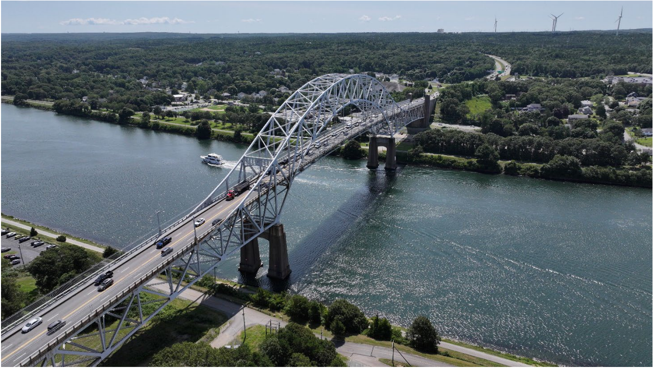
Exhibit 1. View of Sagamore Bridge, facing southeast
