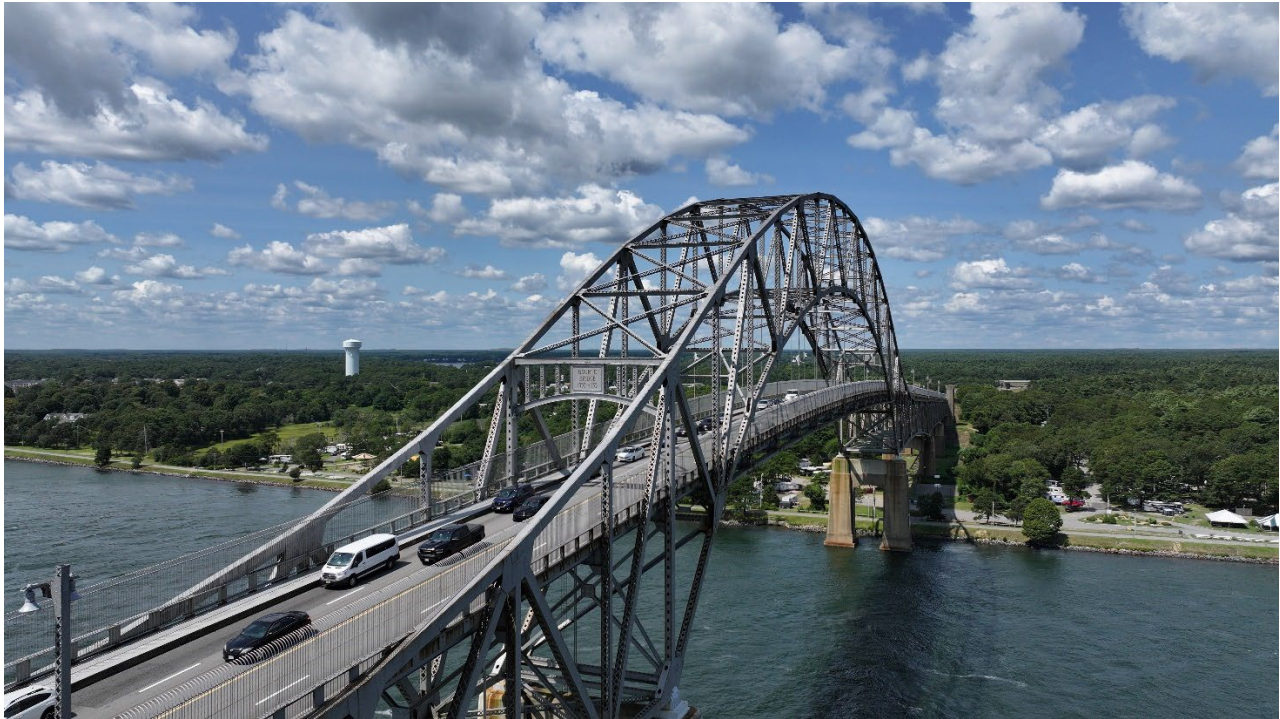
Exhibit 1. View of Bourne Bridge, facing northwest
