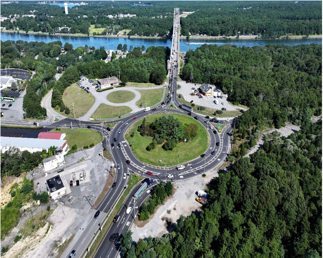
Exhibit 1-4. Bourne Rotary (looking north)
