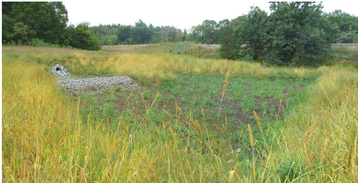
Exhibit 4.10-7. Typical Infiltration Basin with Sediment Forebay
