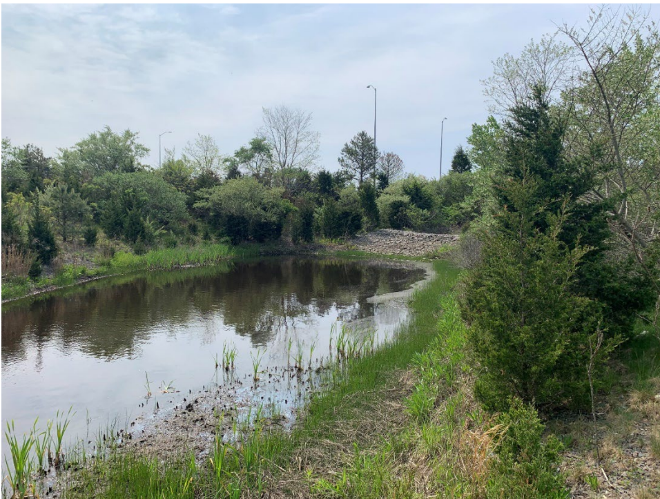
Exhibit 4.10-3. Stormwater Basin at State Route 3 North Off-Ramp (Sagamore North Quadrant)
