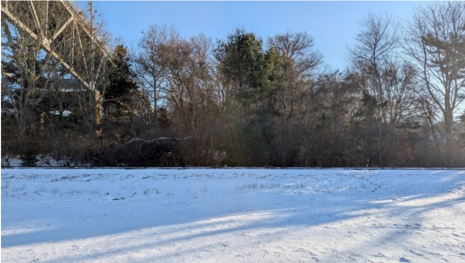
Exhibit 4.15-19a. Existing View of Bourne Bridge from South Canal Service Road, facing south
