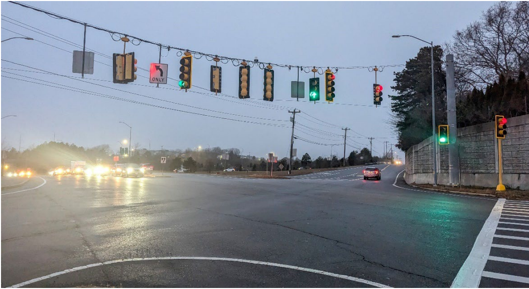
Exhibit 4.15-5a. Existing View of State Road and Scenic Highway from Meetinghouse Lane, facing northwest
