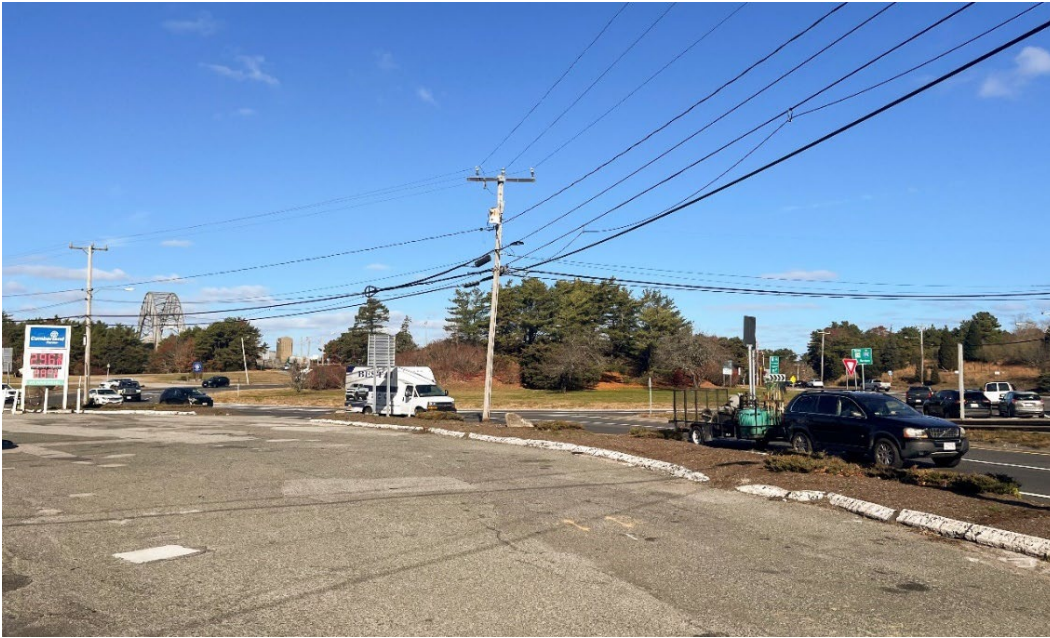
Exhibit 4.15-16a. Existing View of Bourne Rotary from Cumberland Farms Parcel, facing northeast
