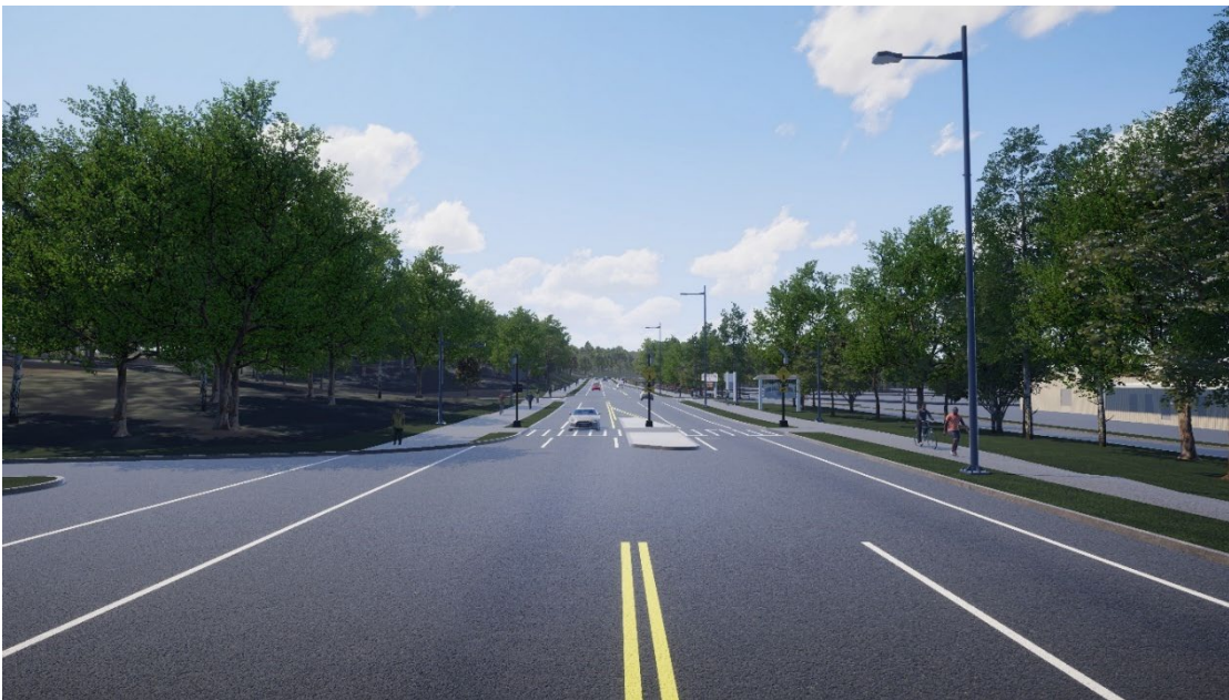
Exhibit 4.15-20b. Simulated View of Sandwich Road at Gallo Ice Arena, facing east
