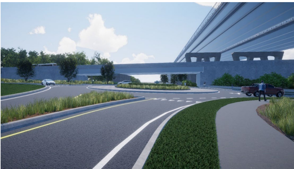
Exhibit 4.15-13b. Simulated View of Bourne Scenic Park from Nightingale Road at Scenic Highway, facing south
