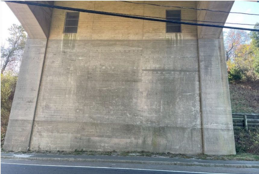
Exhibit 4.15-10a. Existing View of Sagamore Bridge South Abutment from Sandwich Road, facing south
