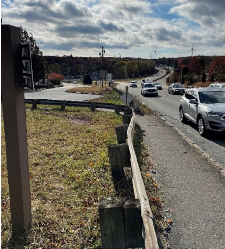
Exhibit 4.3-2. Sagamore Bridge Sidewalk Terminus at Cul-de-Sac (5 Cranberry Highway)
