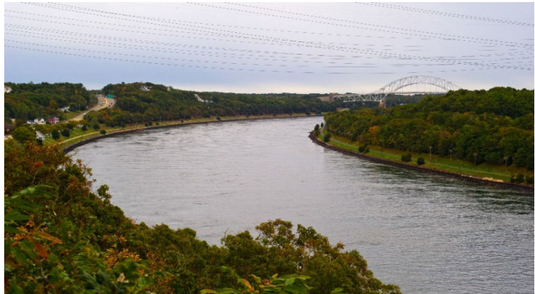
Exhibit 4.4-1. View of Cape Cod Canal, facing east toward Sagamore Bridge, September 2023
