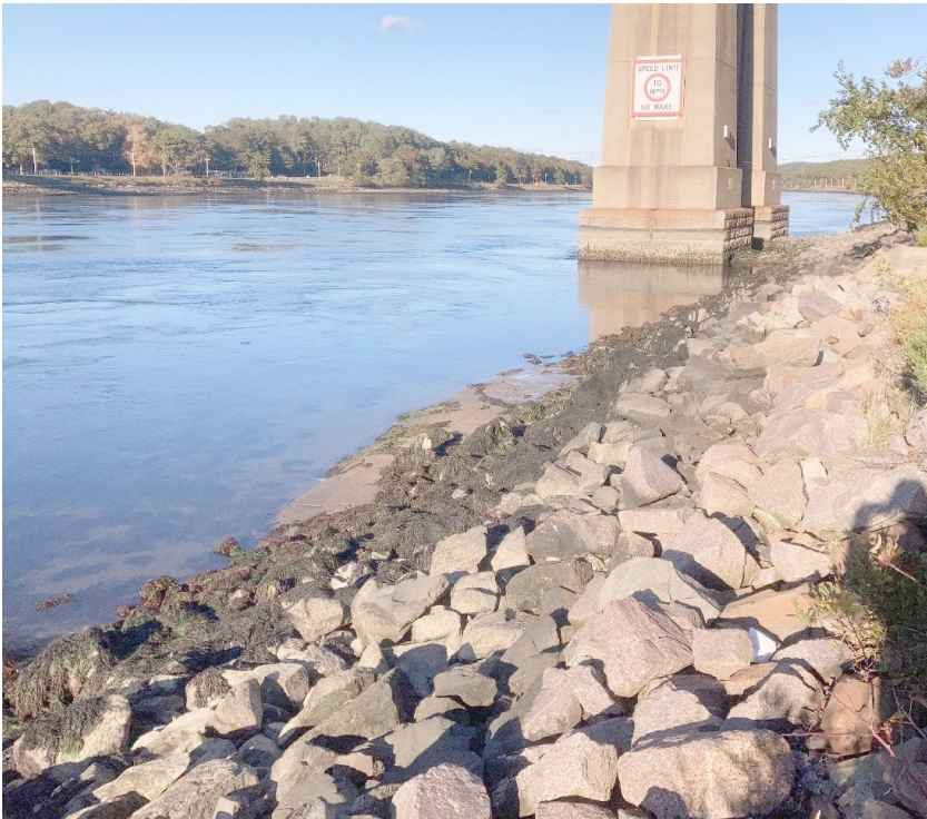
Exhibit 4.9-7. Banks of Cape Cod Canal Adjacent to Bourne South Quadrant Bridge Piers, Looking East
