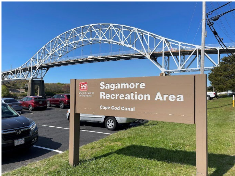
Exhibit 5-1. Sagamore Recreation Area: Sign and Paved Parking Lot, facing southwest
