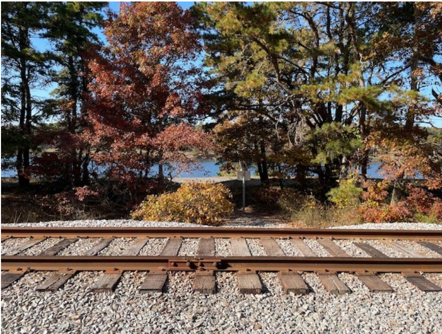
Exhibit 5-33. Railroad Tracks at South Canal Service Road, outside of Arena parcel western boundary, facing north
