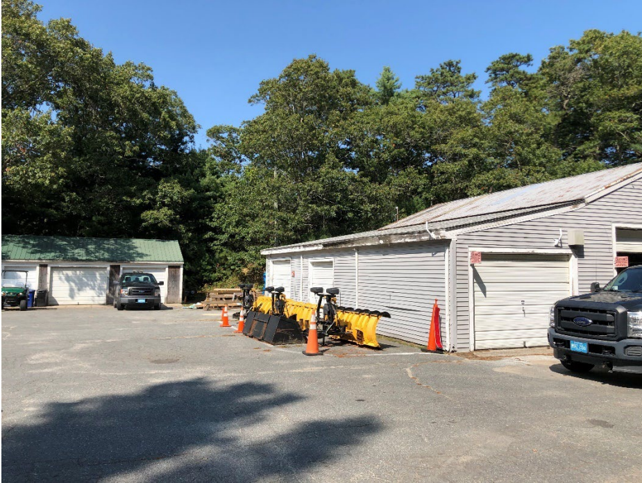
Exhibit 5-12. Bourne Scenic Park: Maintenance Buildings, facing northeast
