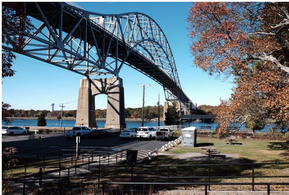
Exhibit 5-23. Bourne Recreation Area: Picnic Tables, Parking, and Portable Toilets, facing north
