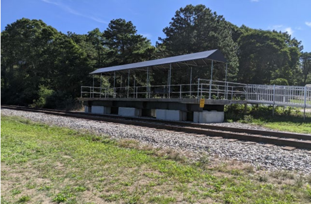
Exhibit 5-26. Bourne Station, facing southeast from South Canal Service Road (outside of Bourne Recreation Area)
