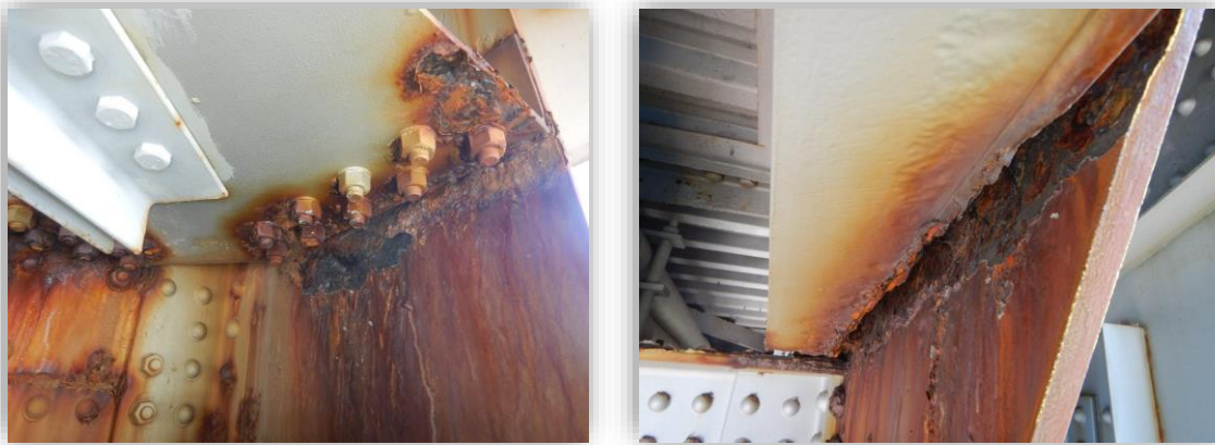
Exhibit 1-1 Photos of Fracture Critical Gusset Plate Deterioration (Bourne Bridge 2020)
