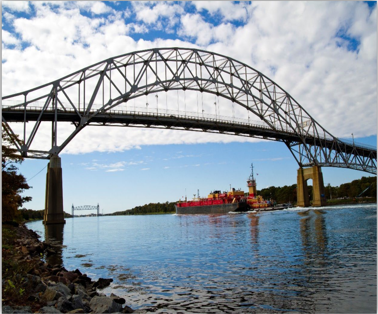
Figure 1. View of the Bourne Bridge looking west towards the Buzzards Bay Railroad Bridge
