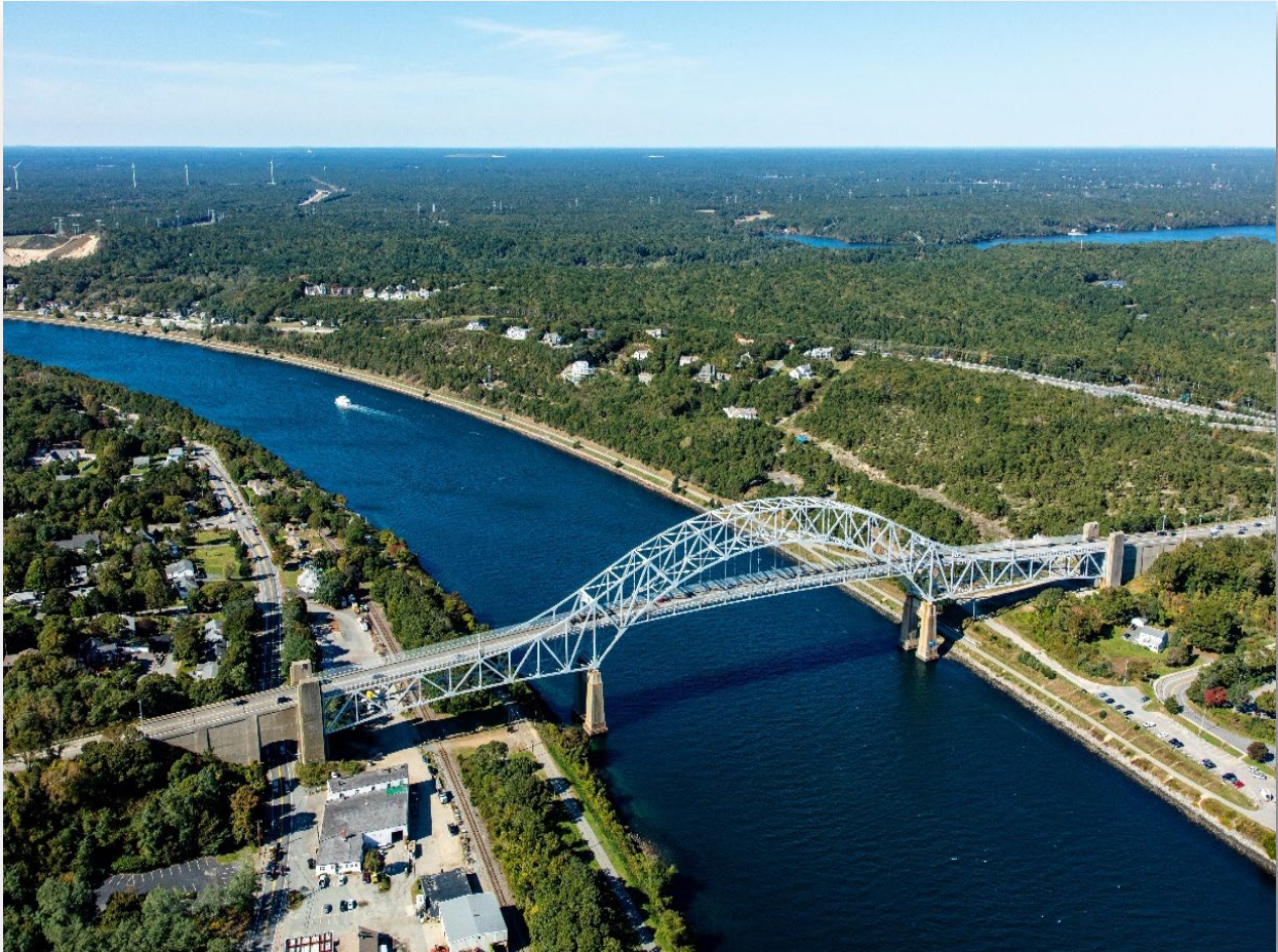
Figure 2. Aerial View of Sagamore Bridge looking west
