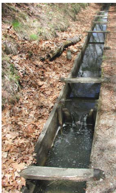
Notched weir-pool fishway at Middle Pond
