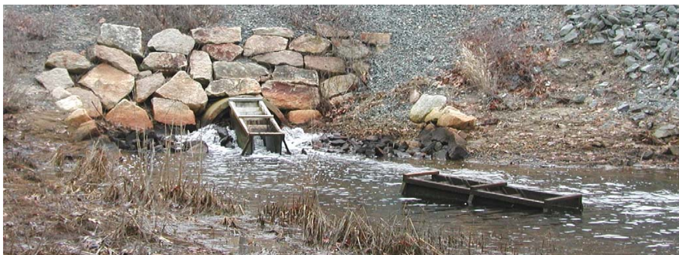
Red Brook Conrail Culvert and Denil fishways
