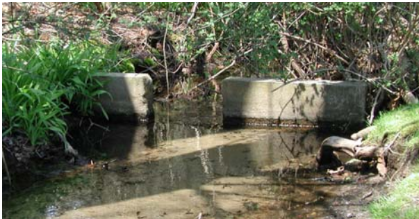
Stream Baffles below Stillwater Lake
