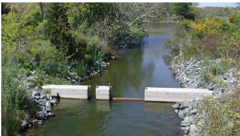
Oyster Pond control structure and fishway
