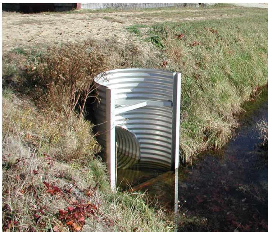
Flax Pond Culvert and fishway
