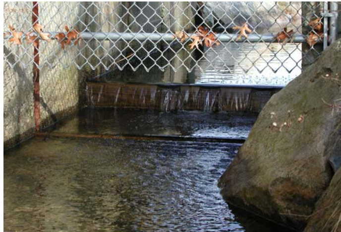
Fishway at Mashpee Pond Control Structure
