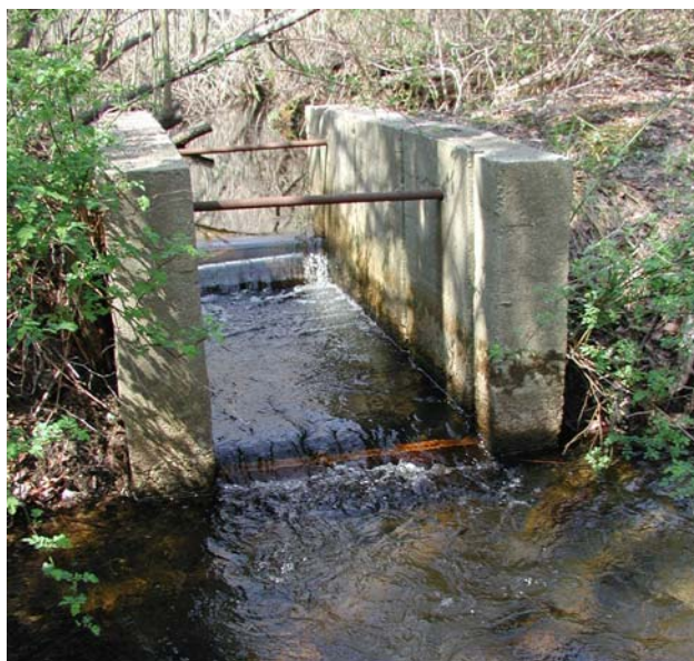
Weir pool ladder at Pond 14 dam (bypassing Alaskan Steeppass ladder)
