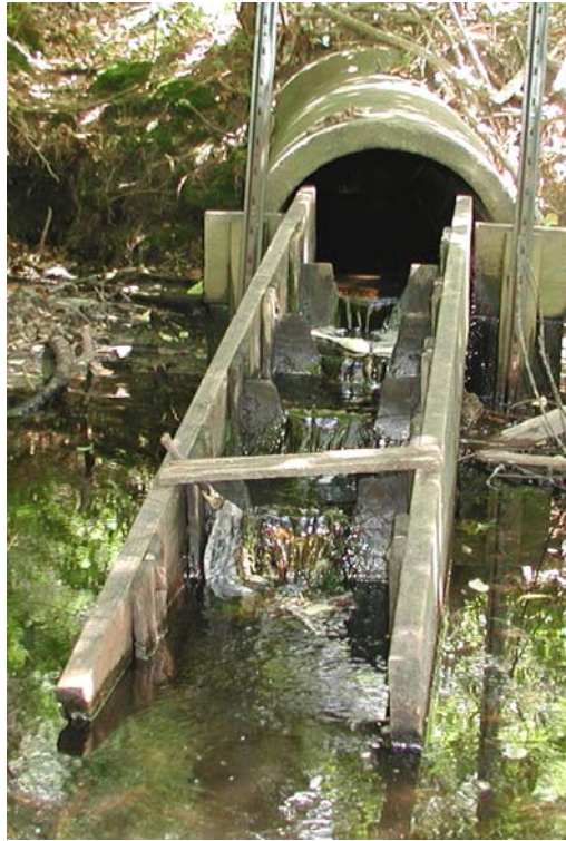
Clear Brook Road Culvert and Ladder
