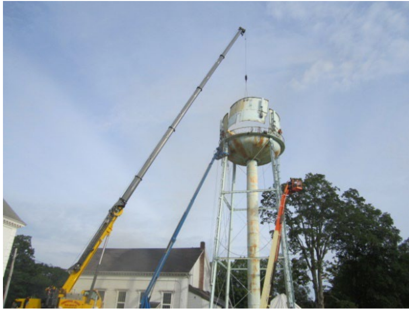
Tank Demolition of the Existing 100,000-gallon tank
