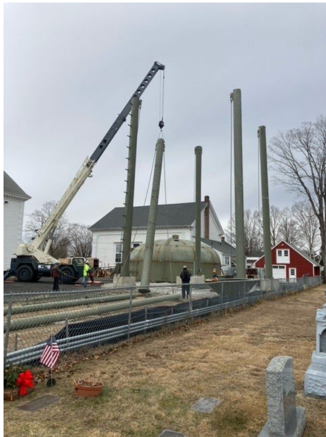
Tank Demolition of the Existing 100,000-gallon tank
