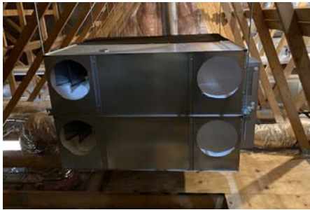
Equipment being installed above library ceiling
