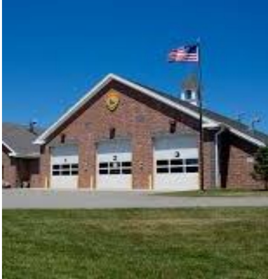
Yarmouth Fire Station 3 – Future Town Emergency Operations Center
