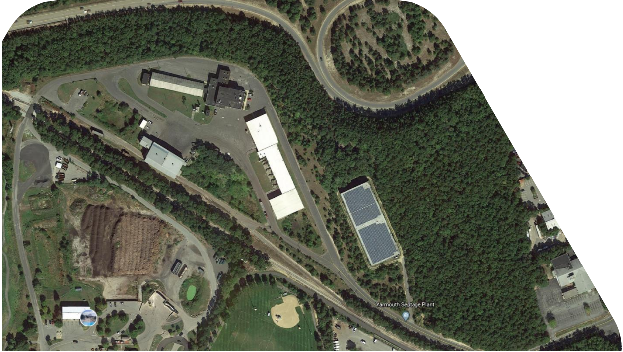
Aerial View of Regional Septic Treatment – Transfer Station Campus
