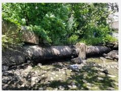
siphon putting both pipes at a greater risk of failure. This will be intensified by increased storm events. Greater installation depths, anchoring, and replenishment of riverbed with native cobbles will protect the siphon.
