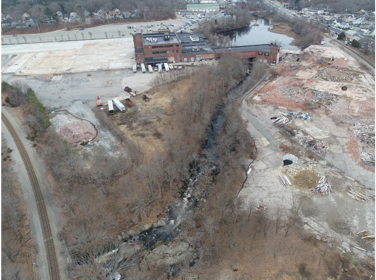
Former Armstrong World Industries Site, December, 2020
