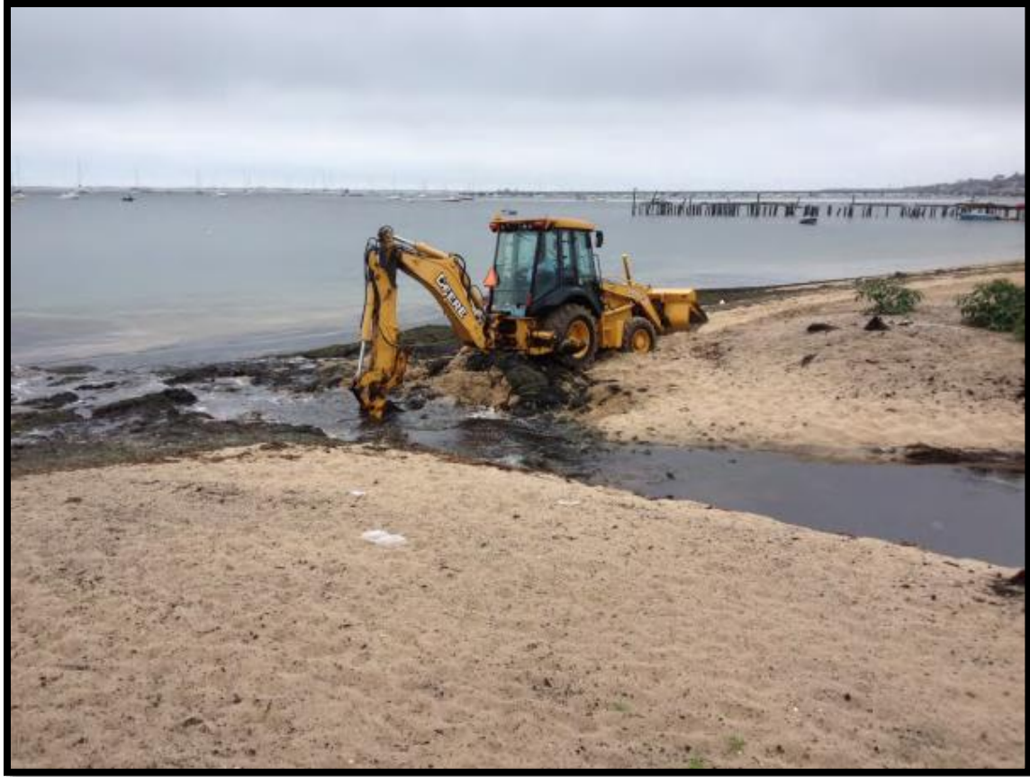
Figure 2 Required Excavation of Outfall during August 28, 2012 Rain Event
