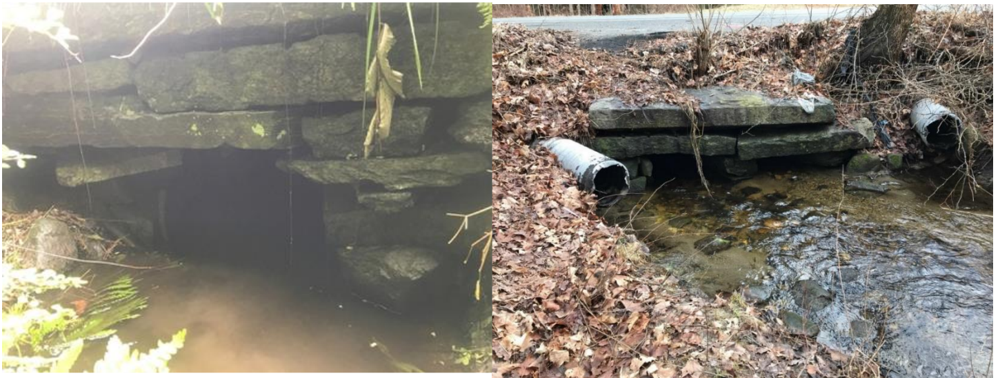
Photos of the inlet and outlet of the Route 181 culvert.
