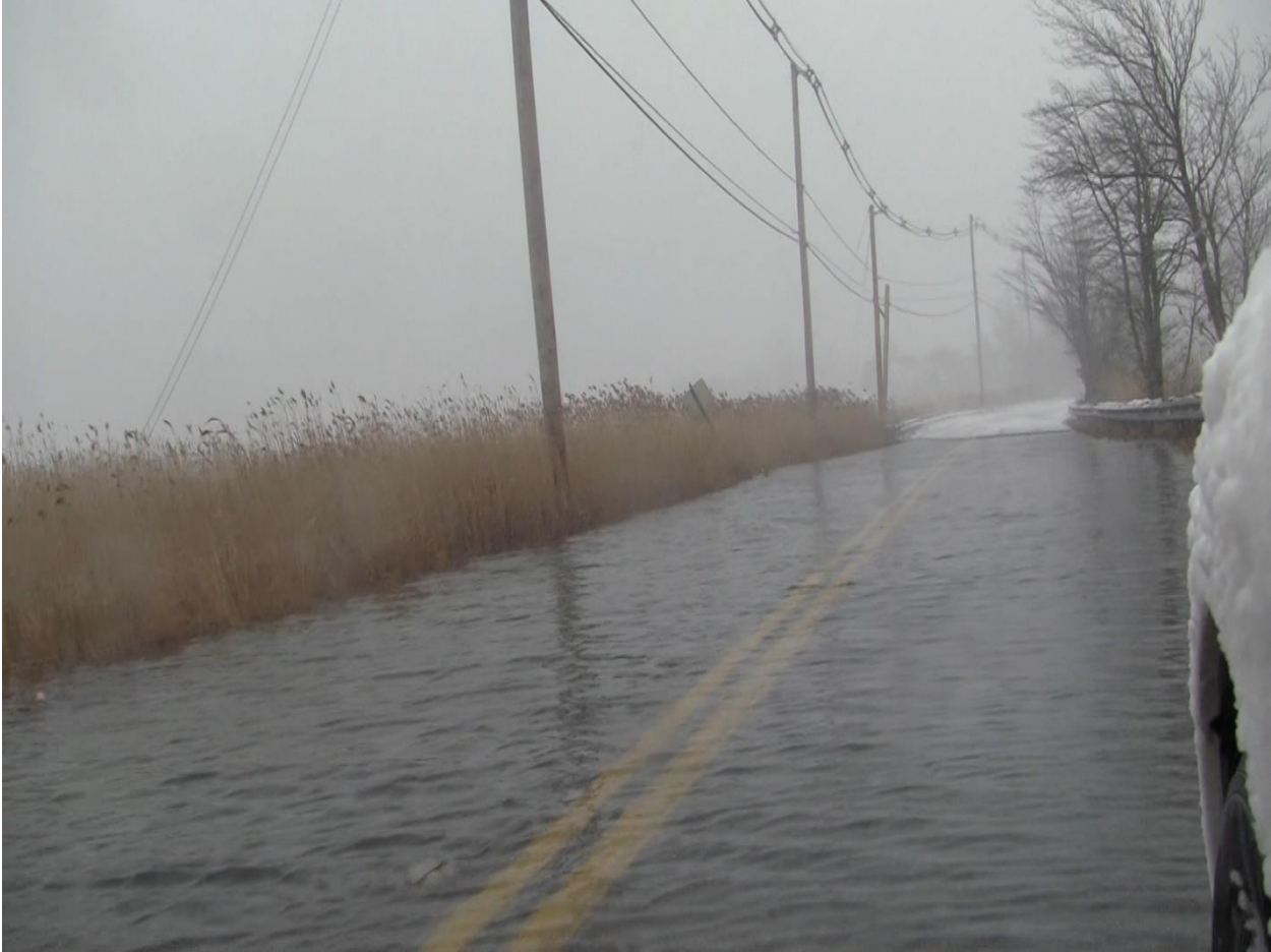
Project Photos: Ferry Road (Photo 1), First Street (Photo 2)
