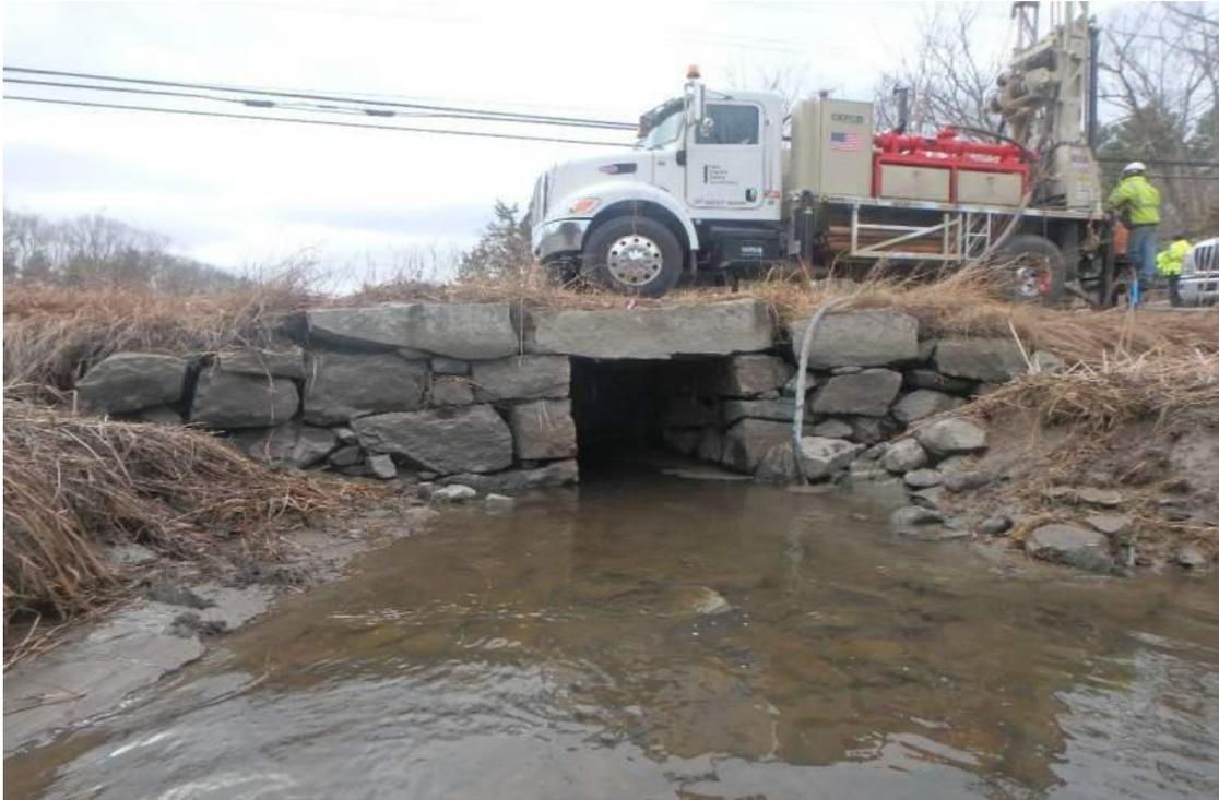
Site assessments and hydraulic analysis determined that a new single span bridge with a 3-sided concrete frame supported by H-Piles would provide the best upgrade at the Orchard Street location. This new structure will supply the benefit of an increased opening width to minimize scour caused by storm events and tidal fluctuations.
