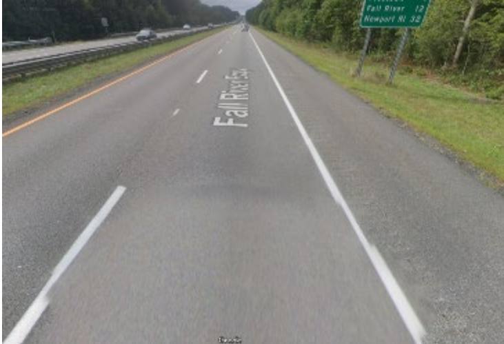
Route 24 Berkley, 2022 Construction
