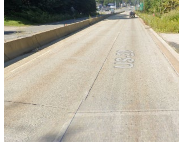
Route 20 Charlton, 2001 Construction
