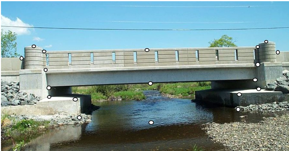
Figure 1.1.5-4b: Single-Span Bridge Survey Locations
