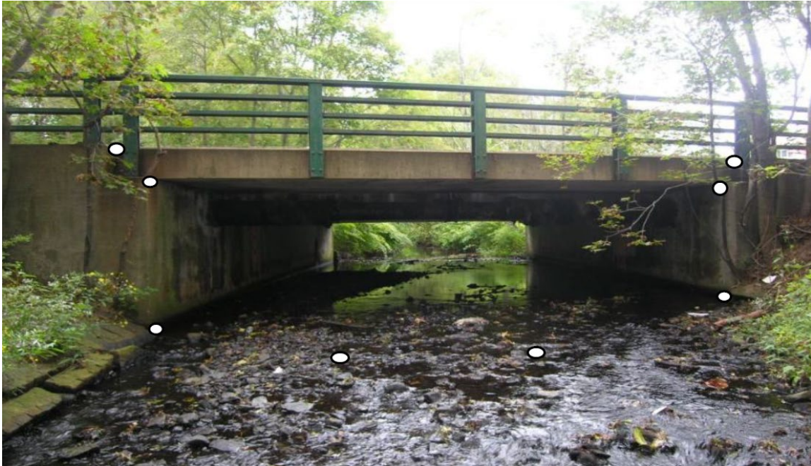
Figure 1.1.5-4a: Single-Span Bridge Survey Locations
