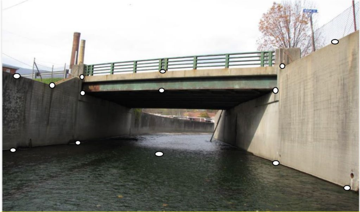
Figure 1.1.5-4c: Single-Span Bridge Survey Locations
