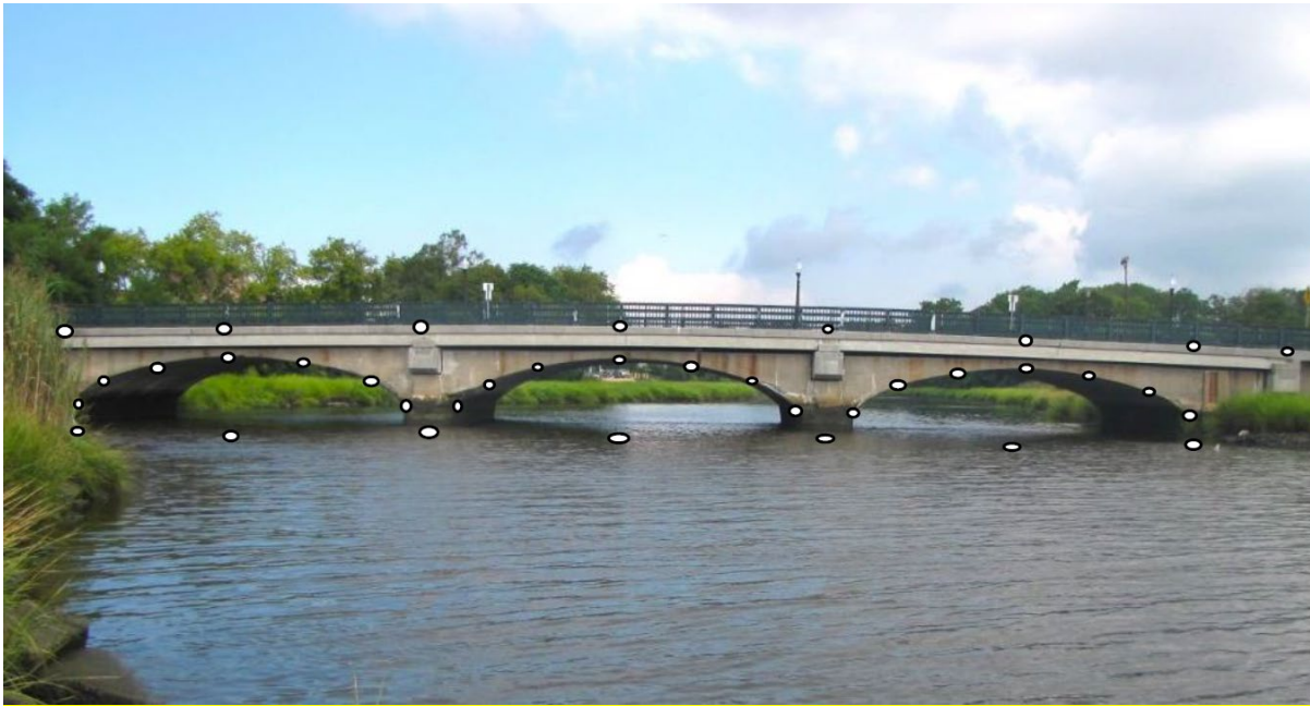
Figure 1.1.5-5b: Multi-Span Arch Bridge Survey Locations
