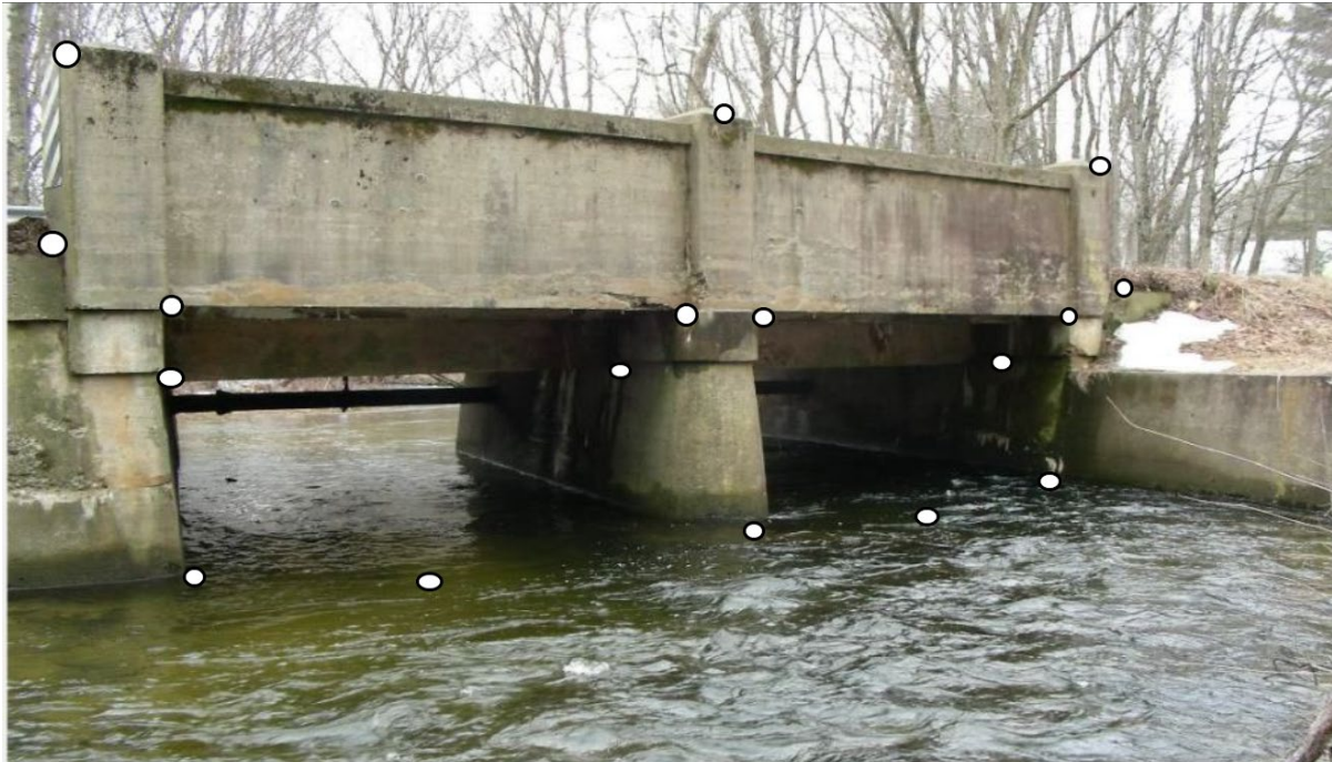
Figure 1.1.5-5a: Multi-Span Bridge Survey Locations
