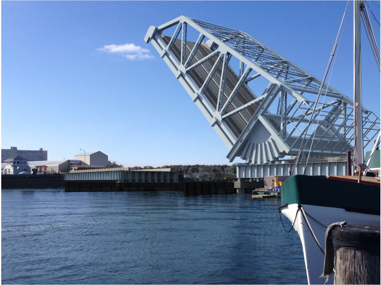
Figure 4.7. Alternative 3: Single-leaf Rolling Bascule Bridge in Open Position
