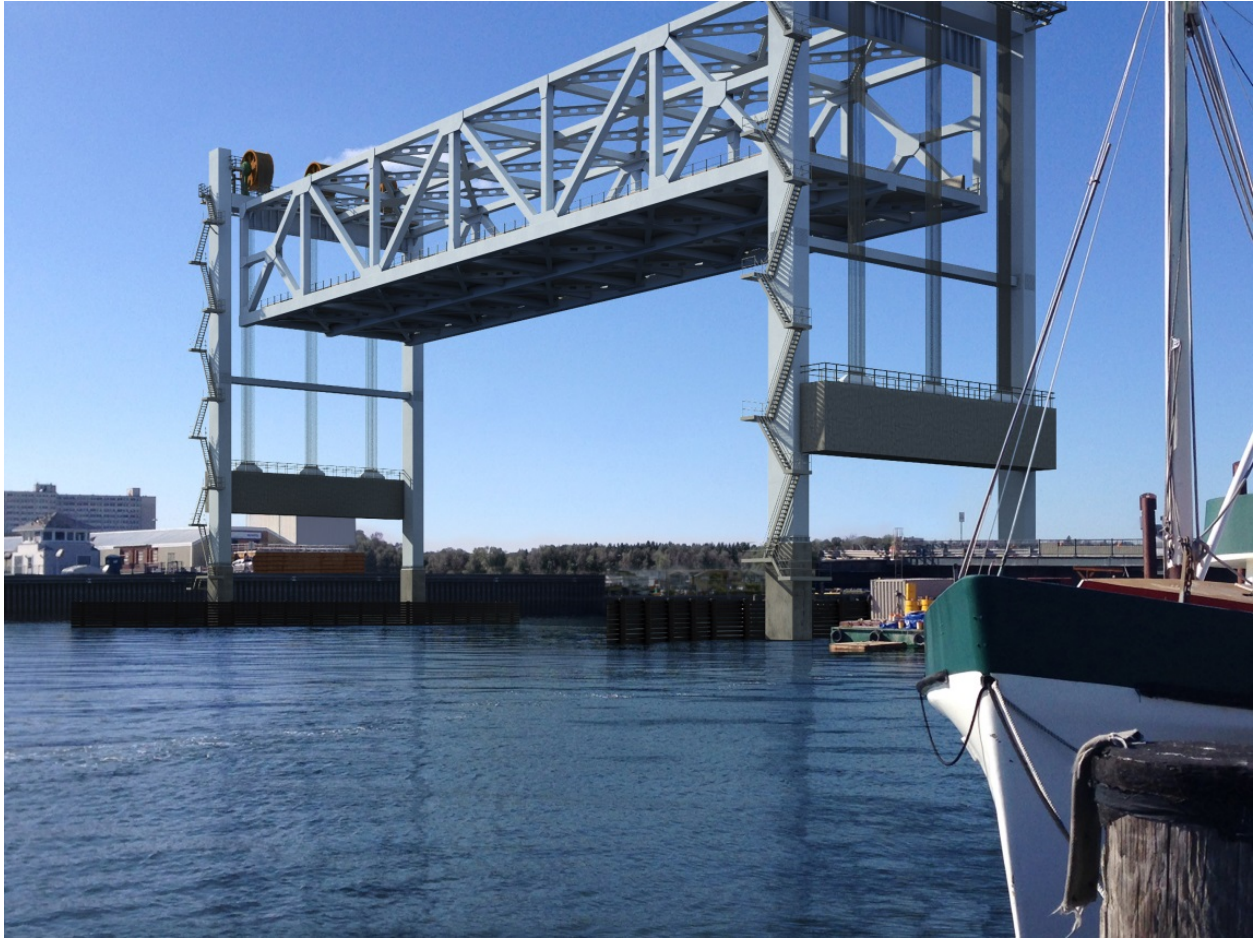
Figure 4.3. Alternative 1: Rendering of Vertical Lift Bridge in Open Position
