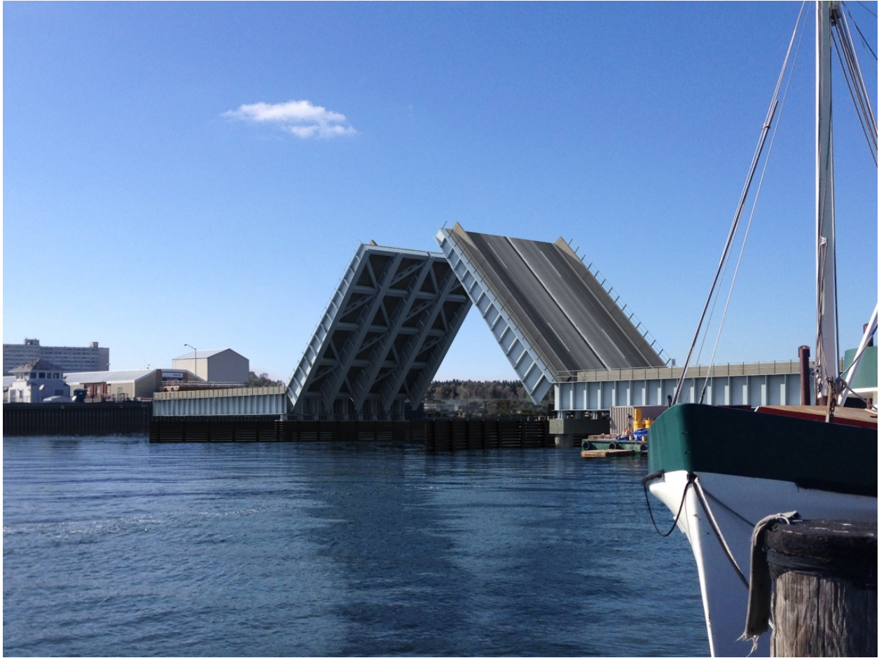
Figure 4.5. Alternative 2: Double-leaf Bascule Bridge in Open Position
