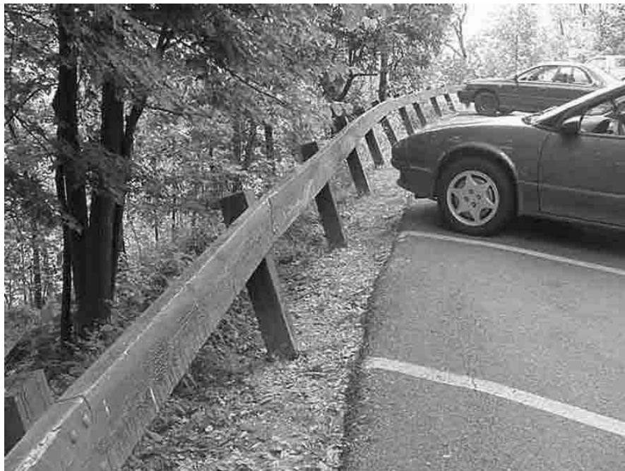
Timber guardrail in Joseph Allen Skinner State Park in Hadley leans from Vehicular impact.
