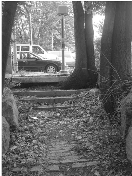
Deferred maintenance along Alewife Brook Parkway now necessitates clearing the path and removing a mature tree to reset the stone step.
