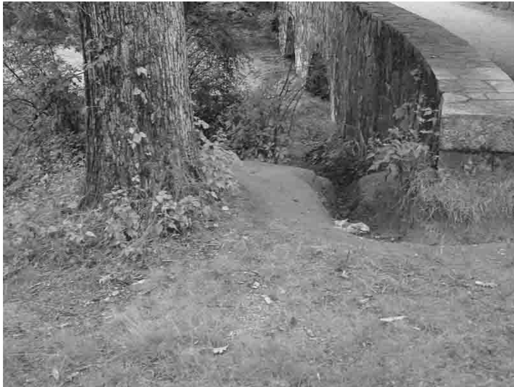
Erosion near the Estate Road bridge at Maudslay State Park in Newburyport requires immediate attention.
