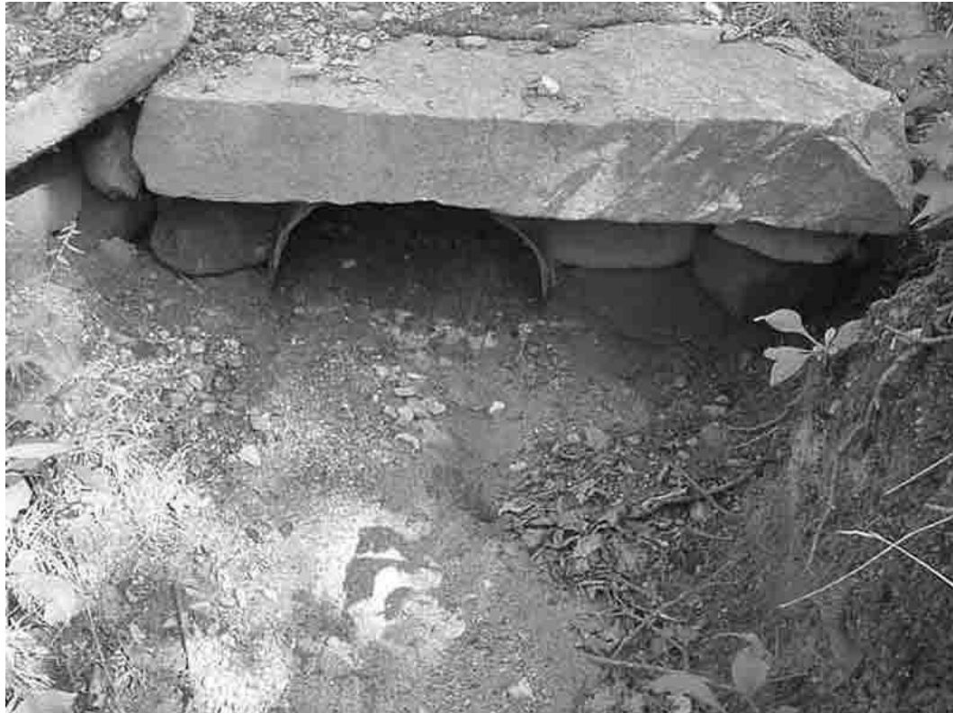
Deferred maintenance on Wickett Pond Road in Wendell State Forest has left the culvert clogged.
