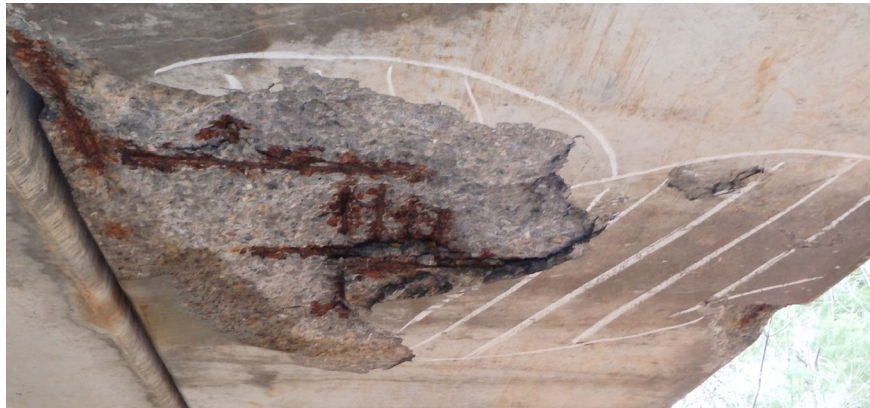
Figure 7.2.10-1: Example of Spalls and Delamination
