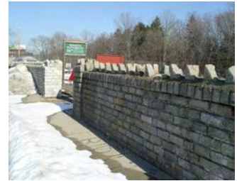
Stone wall along Edgewater Drive at Kennedy Playground
