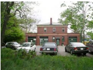
Waterside view of existing Truman Parkway Field Office building
