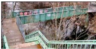
The Glenwood Avenue footbridge provides access across the Neponset River and the MBTA tracks
