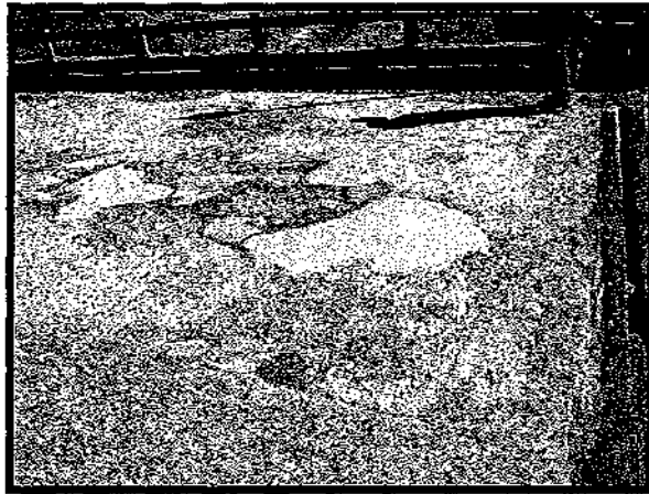
Bridge C-05-010: Deck Deterioration and Failed Joint Seal
