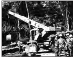
Photo: Army Corps of Engineers
