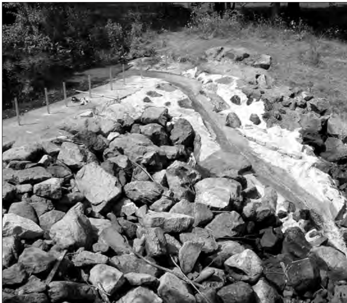
The recently installed chute on the spillway at Woolen Dam in Newbury enables fish migration.
