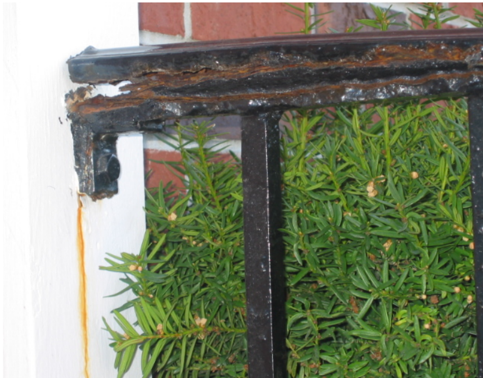
667-1 Development, 228 Crowell Road Unsafe and Rusted Front Door Railings
