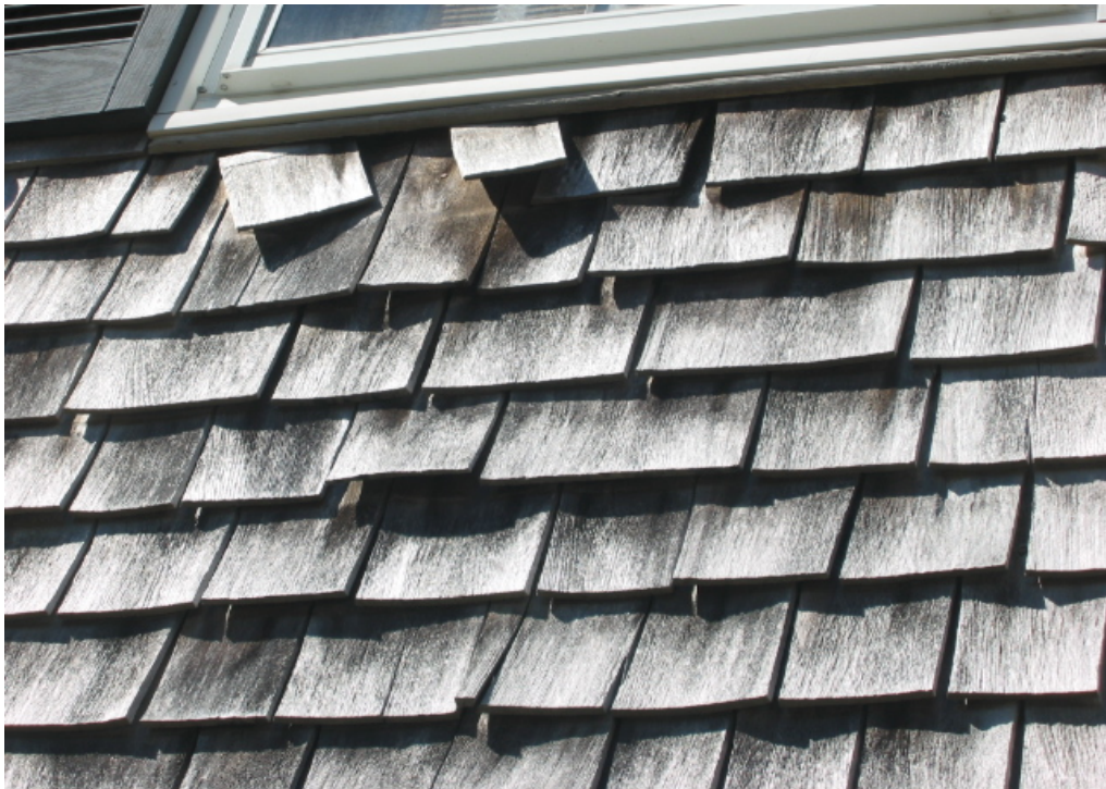
667-1 Development, 256 Crowell Road Shingles Falling off Building
