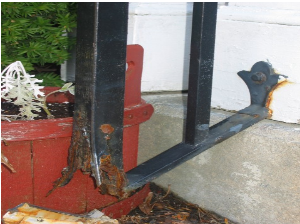
667-1 Development, 256 Crowell Road Unsafe and Rusty Stair Railing
