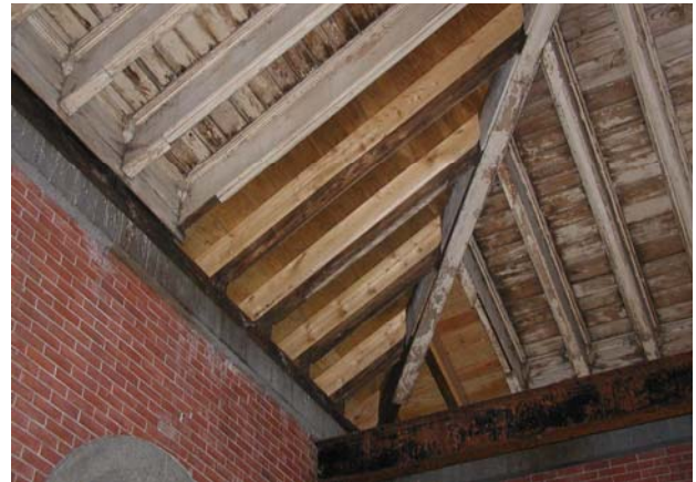
Figure 3.9: Modern materials in southwest corner of roof (2005)
