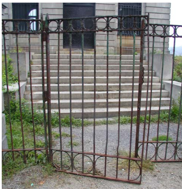
Figure 3.33: Gatehouse #2 gate with missing circular elements (2005)
