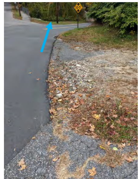
Photo 7-2: Loose sediment along the eastern shoulder of Elm Street.
