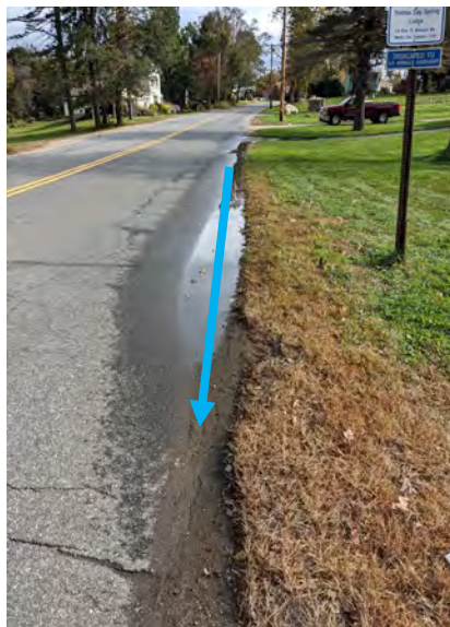
Photo 11-2: Ponding in the shoulder along Wilbraham Road.
