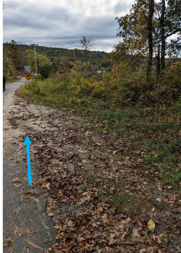
Photo 13-2: Dirt pull-off eroding and washing into adjacent wetland.
