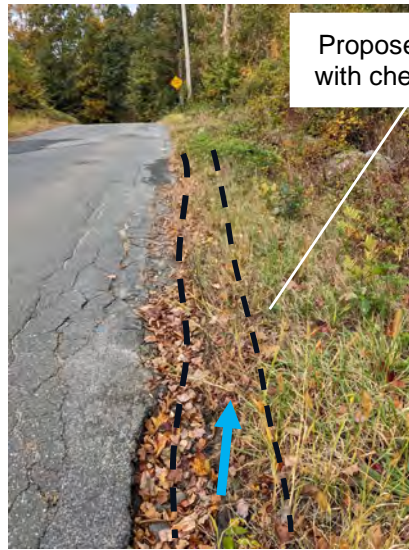
Photo 9-2: Erosion along the shoulder of Carpenter Road.
