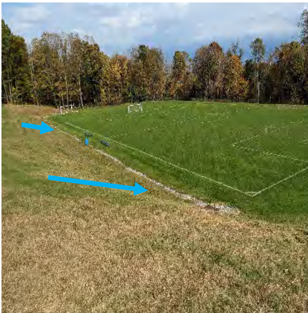
Photo 12-1: Existing French drain along upgradient side of field.
