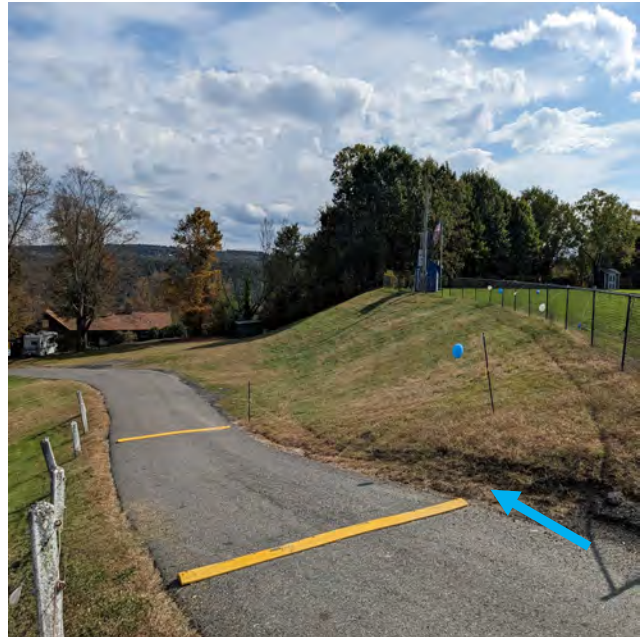
Photo 12-2: Shoulder erosion along the paved access roadway.
