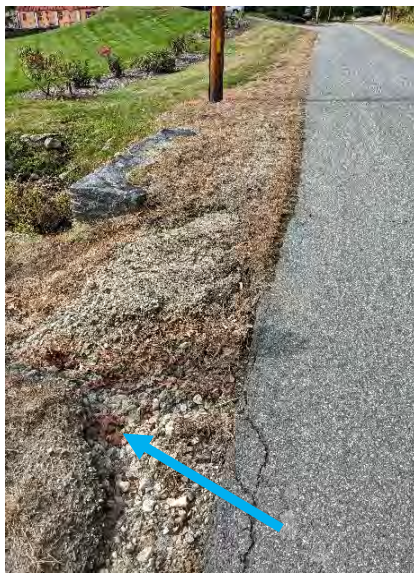
Photo 11-1: Erosion around the culvert.
