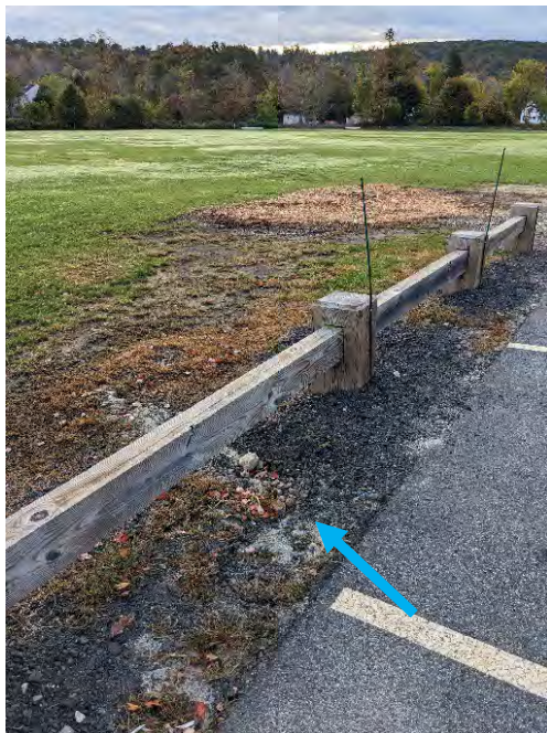
Photo 4-1: Erosion around the parking lot.
