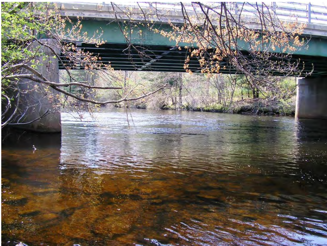
Figure 8 Station WA09A upstream (4/28/2009)
