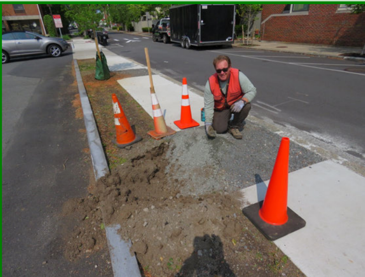
DCR Forester Dave Bresnahan using structural soils to improve tree growth in Salem.
