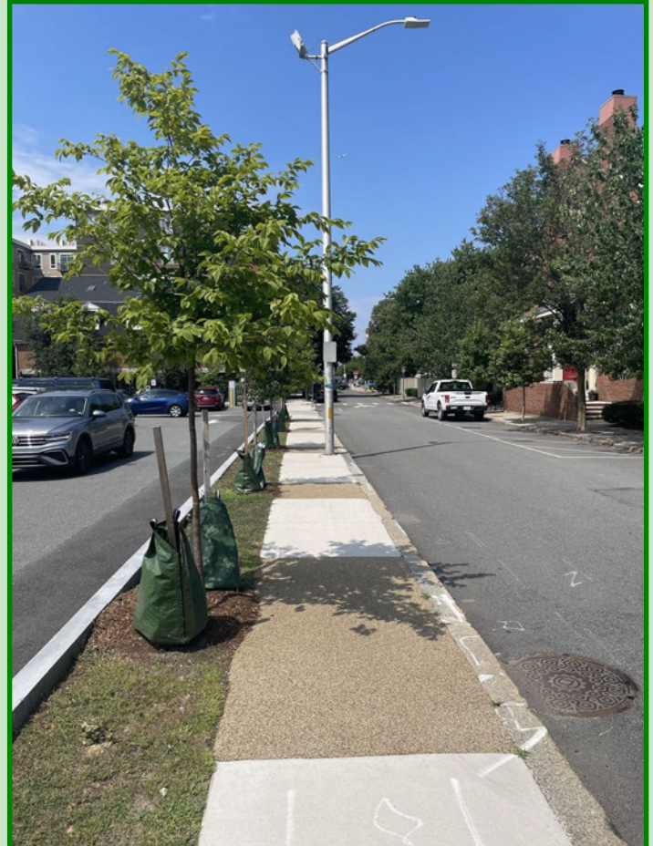
Completed Salem project including a flexi-pave sidewalk covering.
