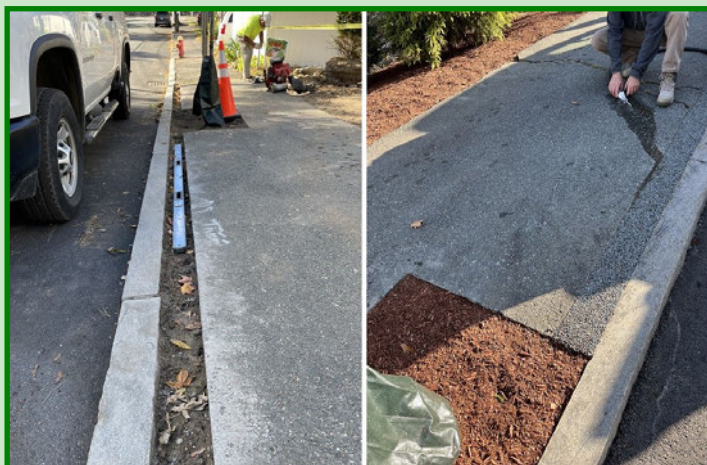
Before flexi-pave installation (left) and after installation with water capture demonstration (right). Photos: DCR
