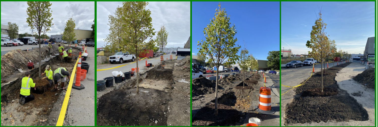
DCR Everett crew plants an industrial lot just outside of Rivergreen Park in Everett. A trench 150'L x 7'W x 3'D was removed and replaced with soil, and DCR installed nine trees.
