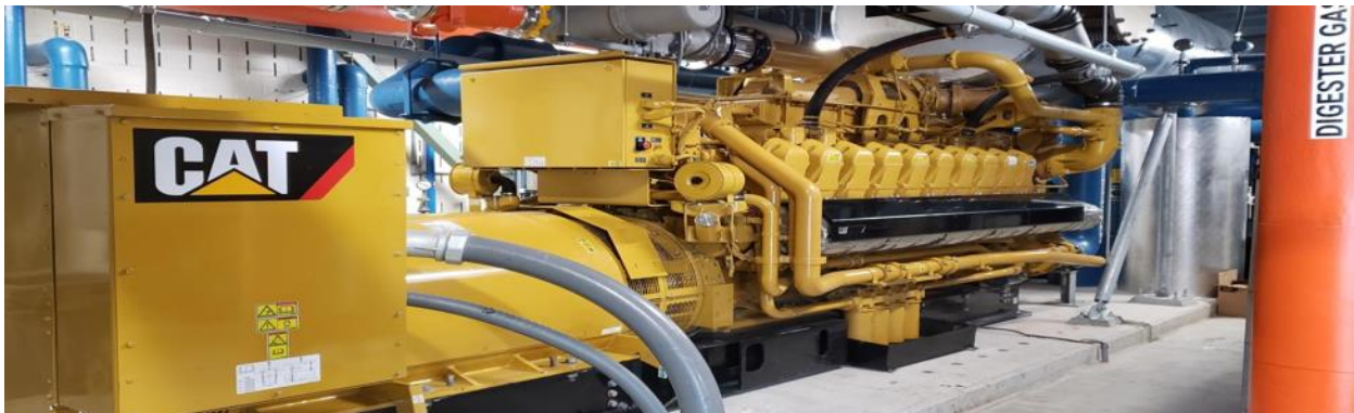
One of two 1.6-Megawatt Caterpillar G3520C co-generation engine.
