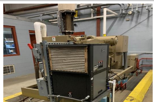
Heat pump for emergency generator
