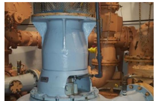
Rebuilt Return Activated Sludge Pump
