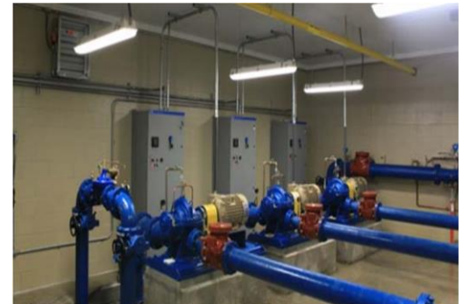
New Jarry Drive PS pumps and controls
