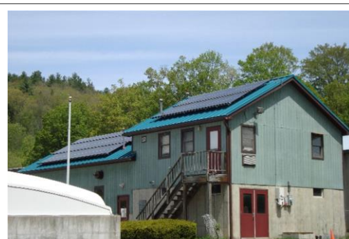
11.7-kilowatt rooftop solar array
