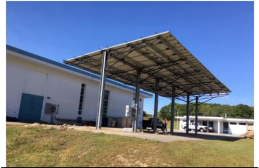
25-kW solar PV carport
