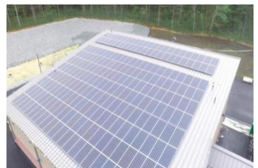
84.3 kW solar PV array
