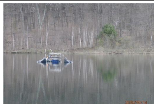
Solar-powered mixer in Root Reservoir
