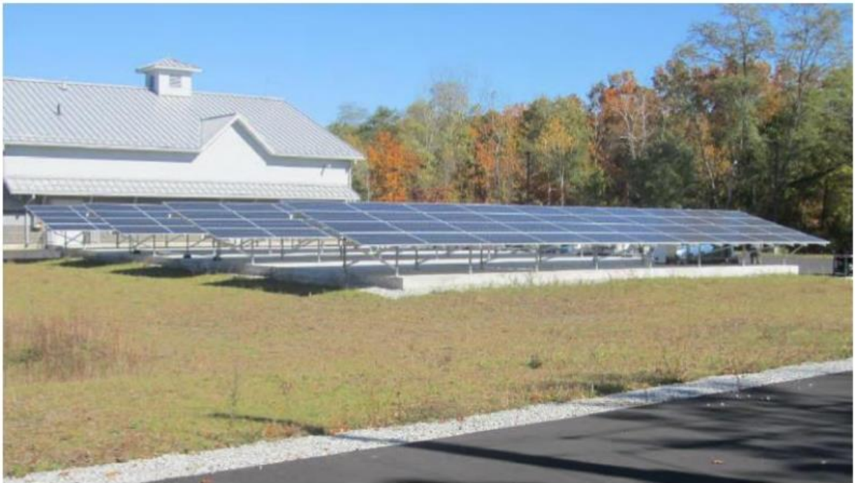
Town of Shrewsbury 59-kilowatt (kW) solar photovoltaic system Home Farm water treatment plant
