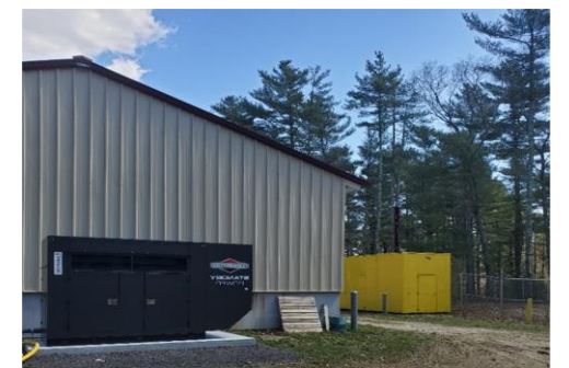
New 125-kW propane generator
