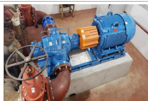
10-kW hydropower pump as turbine
